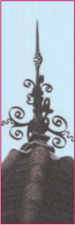
Ornate ironwork finials.
