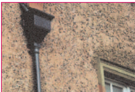
Original cast iron hopper and downpipe
