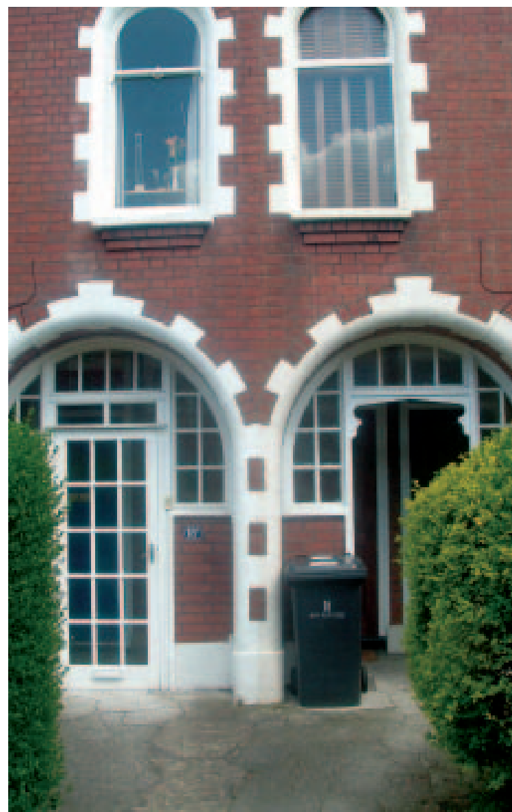
Fig 18: Inserted door in outer timber panel screen
