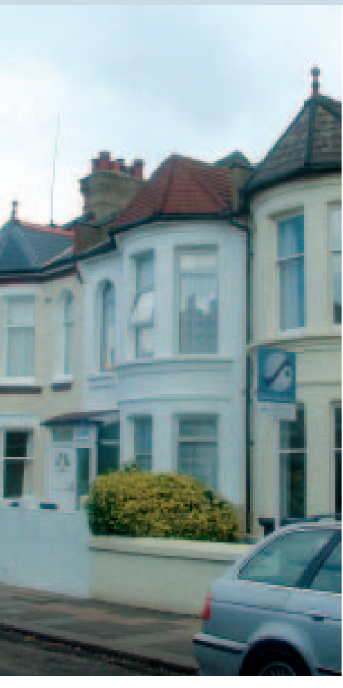
Fig 13: Rendered brickwork
