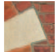
Fig 8: Fine pointed facing bricks
