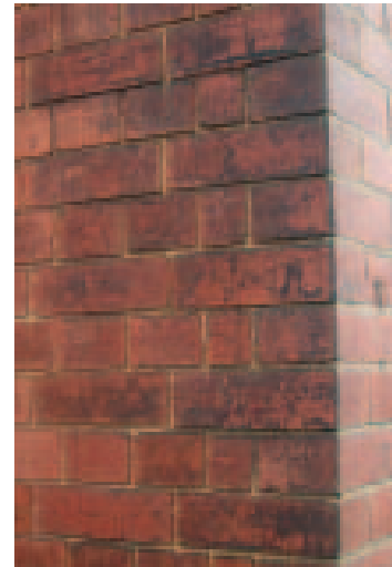
Fig 8: Fine pointed facing bricks
