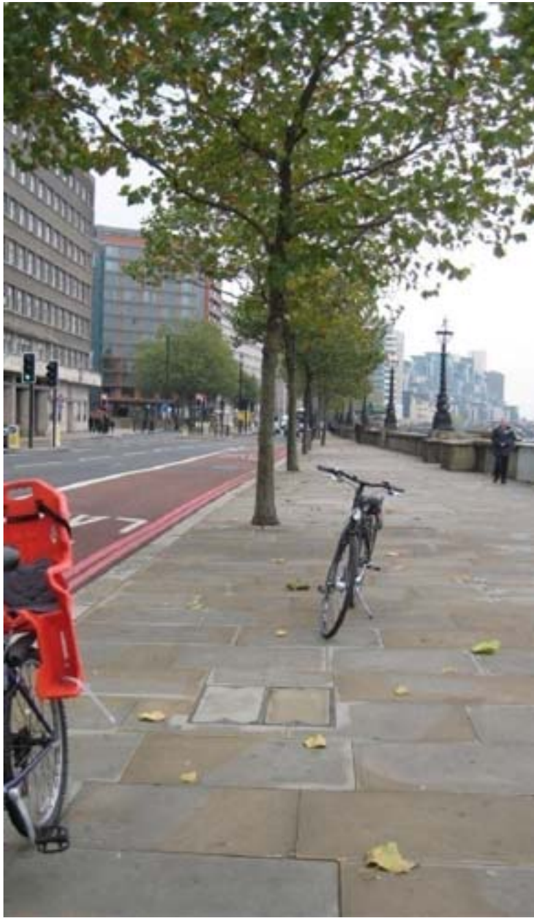
49. Fire Brigade Pier (Albert Embankment)
