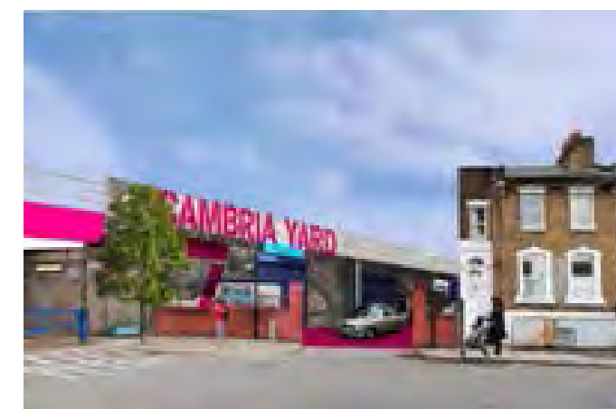
Cambria Yard, adjacent to Cambria Bridge
