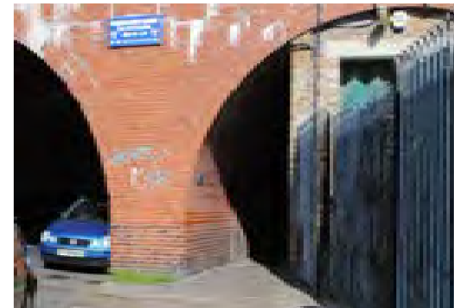
(a) Gordon Grove pedestrian access Unpleasant passage under bridge; poor lighting; restricted access for passing pedestrians
