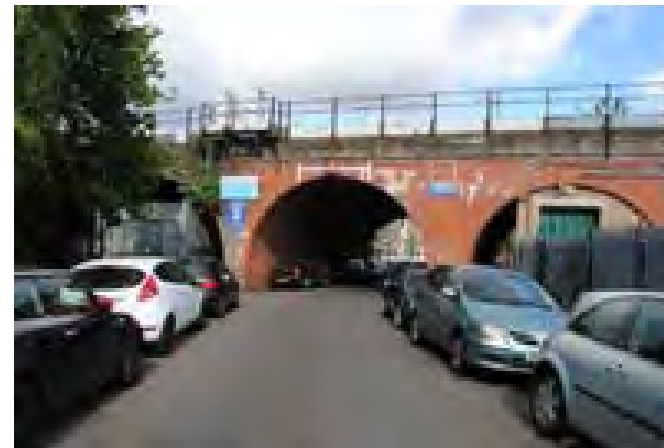
(a) Gordon Grove railway bridge Restricted view; restricted access for passing vehicles; no alternative for cyclists
