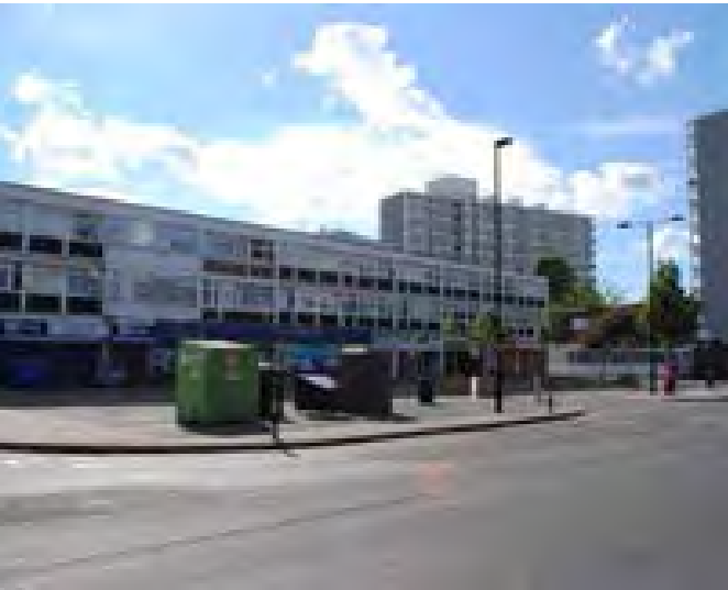
Existing view from Loughborough Road
