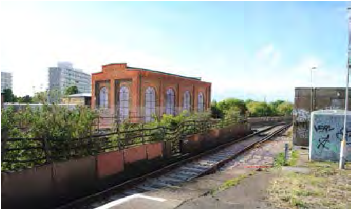
Proposed refurbishment of substation (still in use) as new public building
