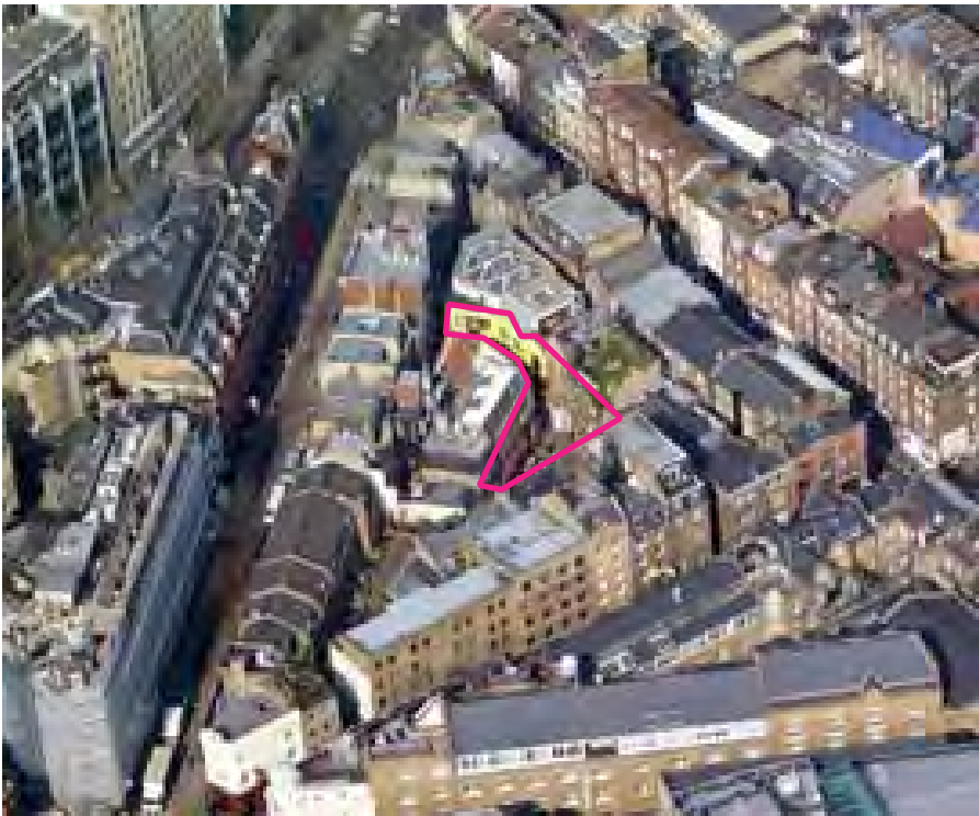
Neal's Yard, Camden WC2
