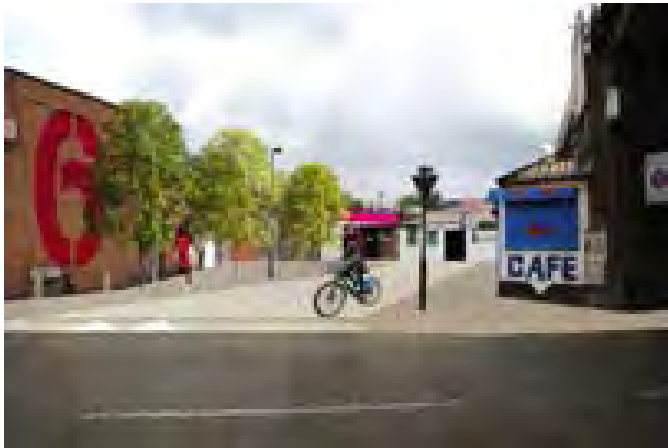
Highways and public realm improvements to Padfield Road
