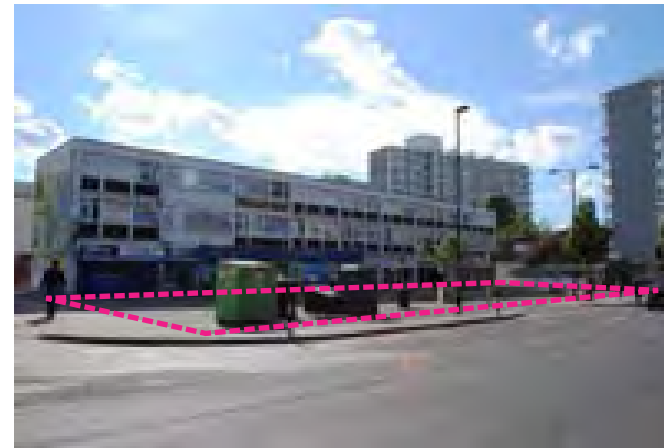
(ii) Public space on Loughborough Road
