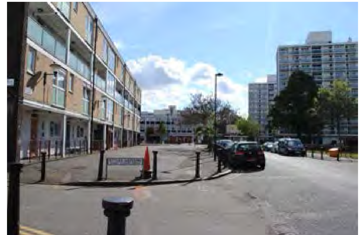
Underused public space on Minet Road - Gateway to Styles Gardens
