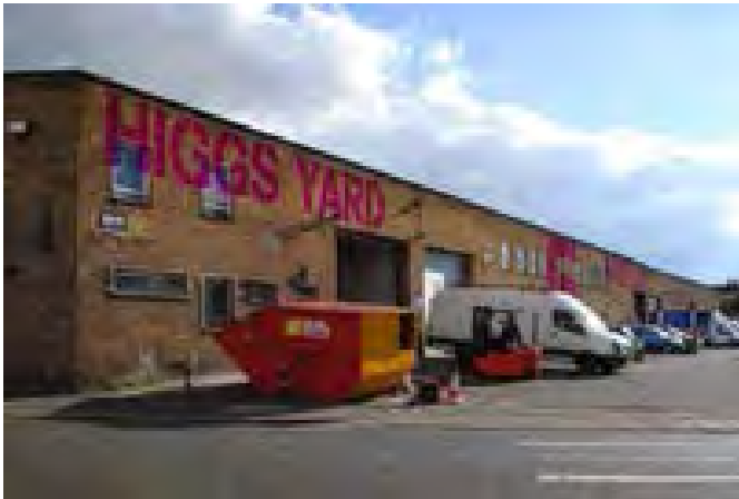
Building the identity of Loughborough Junction through coordinate signage and wayfinding
