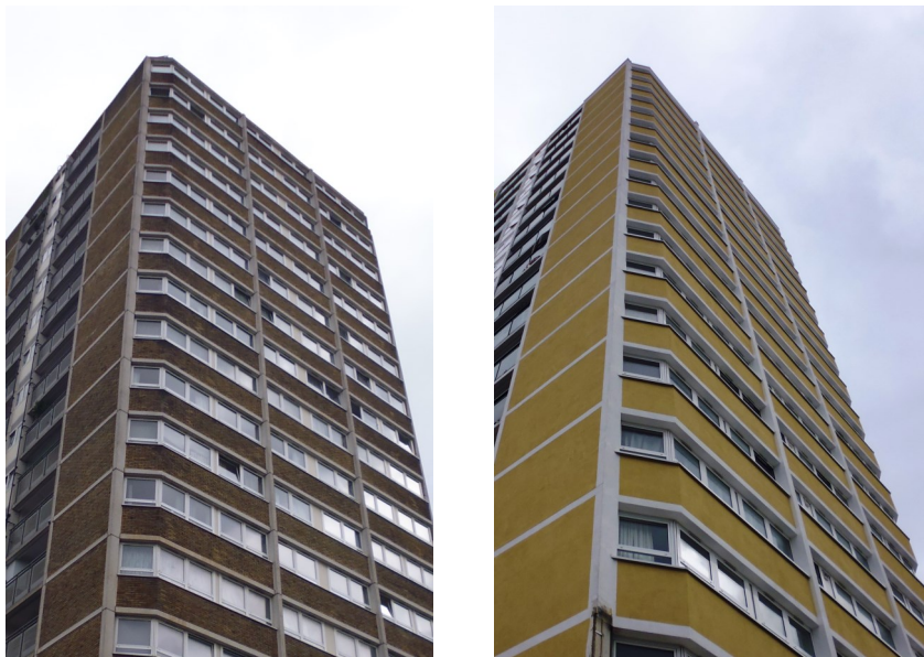
Before and after: the application of external insulation has successfully respected the architectural character of this tower.
