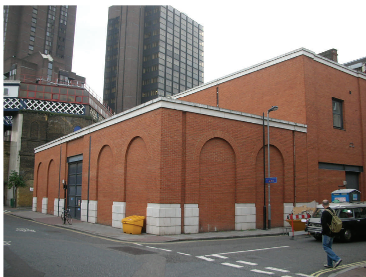
London Underground tube shaft building, Alaska Street
