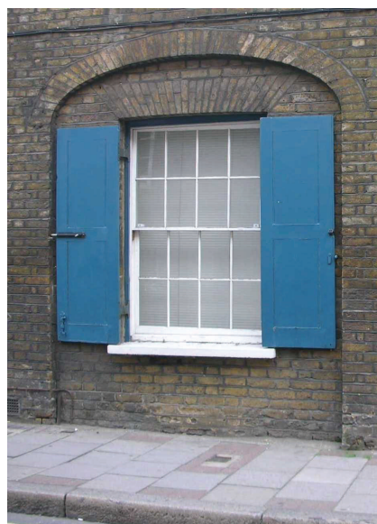
25 Cornwall Road has the only surviving shutters.
