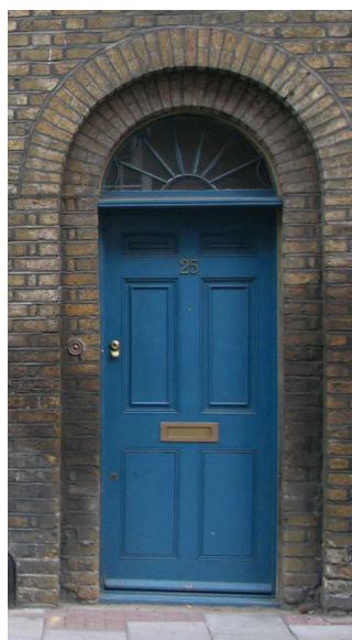
Historic doors should be retained.
