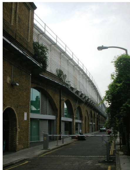
The railway viaduct, Brad Street
