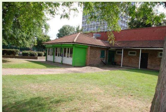
Existing café building.
