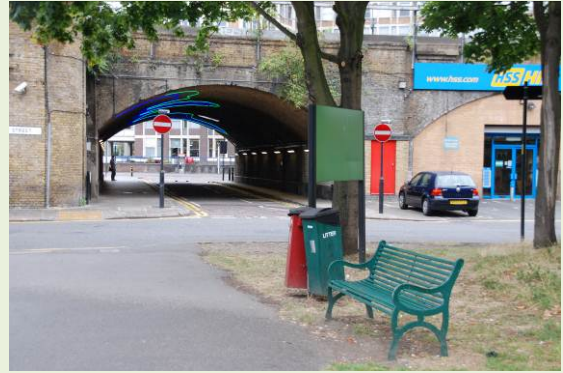
Archways beneath the railway viaduct.
