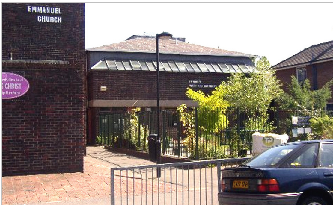
Emmanuel Youth Centre. The £15,000 Youth Facilities Contribution from the former St Saviours College site Gipsy Hill paid for improvements to The Emmanuel Youth & Community Centre which required upgrading of the electrical wiring and fire safety equipment. The Centre is a purpose built facility that serves residents of the local community.
