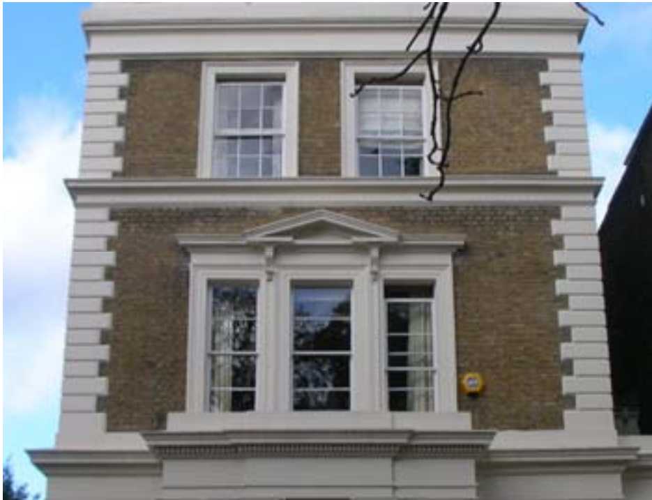
Fine stucco detailing is an important feature of the Albert Square houses.
