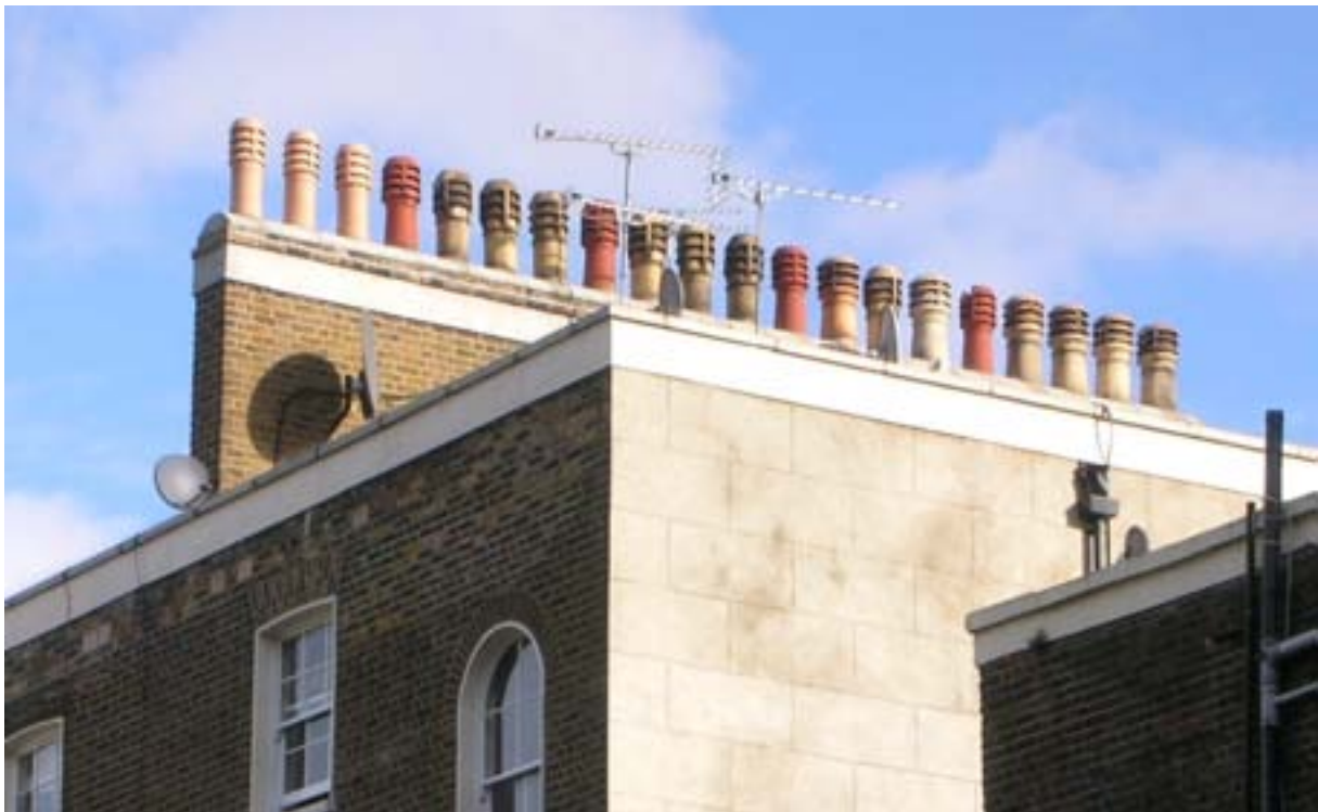
Brick chimney stacks with terracotta pots are an important feature of the conservation area.
