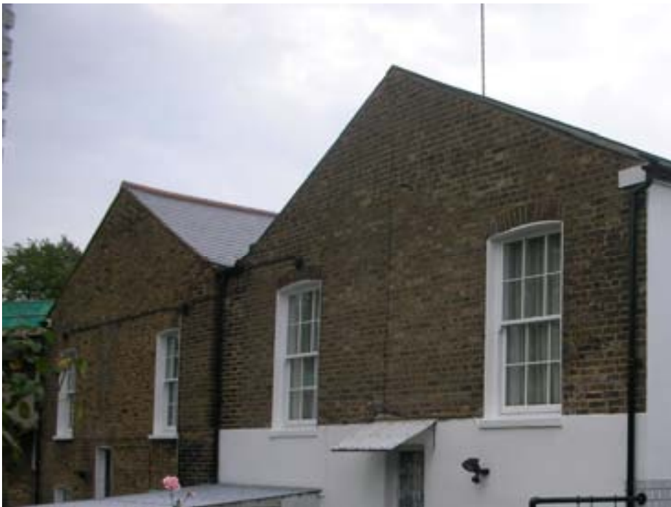
Roofs should be naturally slated and devoid of clutter.
