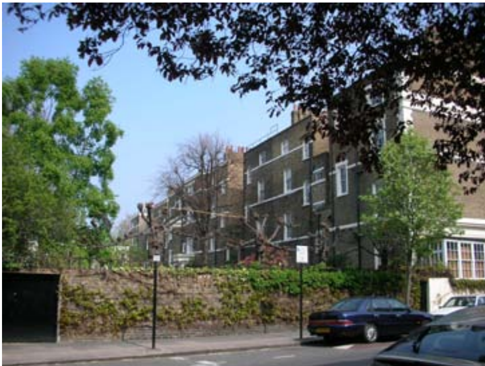
Some views of rear elevations are particularly prominent and important.
