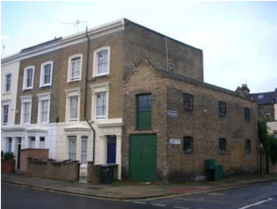
This little commercial building adds interest to St Stephen's Terrace.
