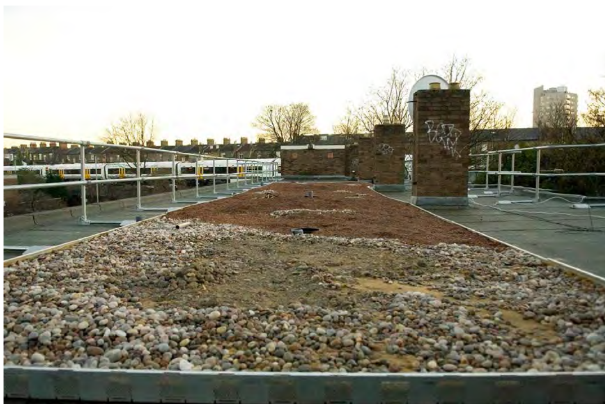
Plate 60. A new biodiverse living roof being constructed on the Fenwick Estate in Stockwell; the close proximity of a network of railway lines, as seen in the distance, was a key reason for its installation in order to extend and improve wildlife habitat
