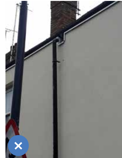
Poorly executed external insulation
