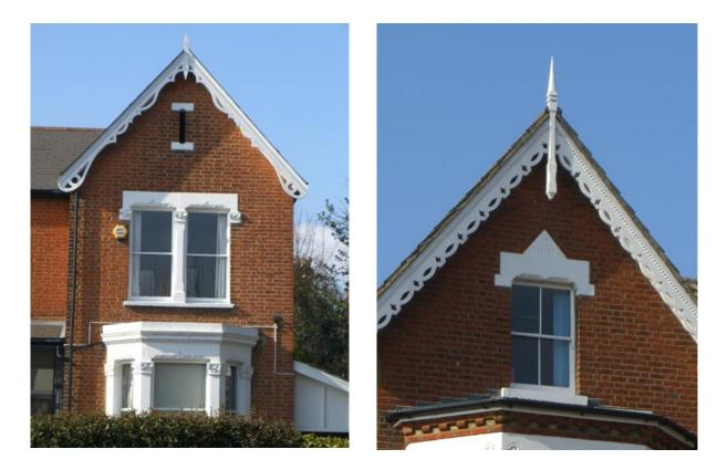
Sash windows with a 1/1 configuration (left) and 2/2 configuration (right) are common.
