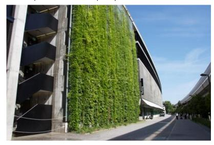
An example of a green wall using climbing plants on strained/tensioned wires.
