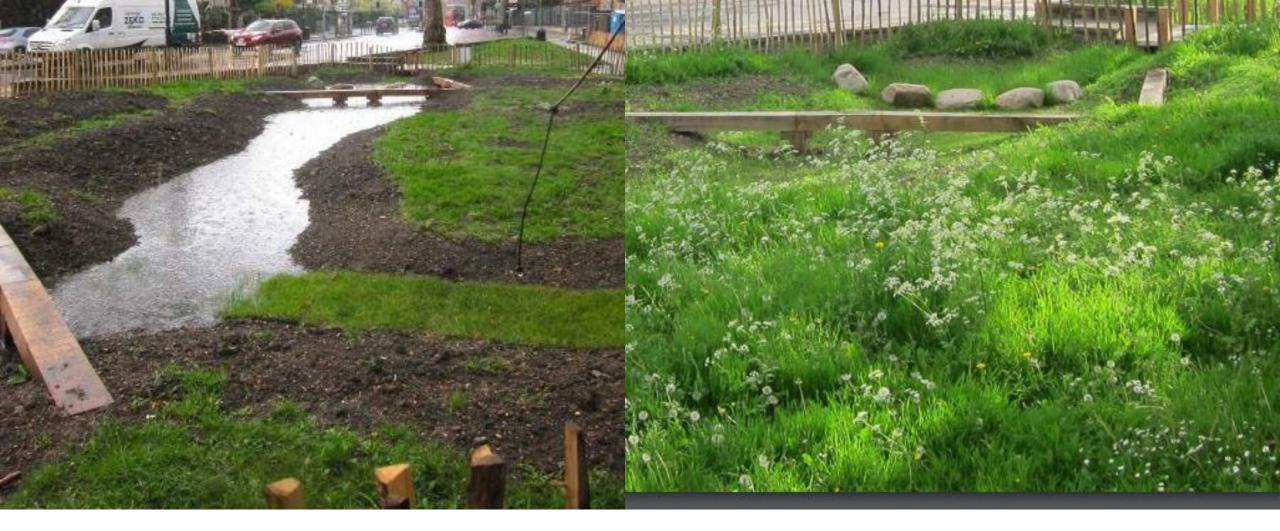
A swale or rainpond, is a landscaped scoop, or series of scoops in a grassy area, designed to collect rainwater from surrounding surfaces. The water is held as a temporary pond – sometimes wet, sometimes dry.
