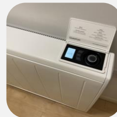
HHR smart storage heaters
