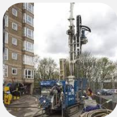
Shared ground loop heat pumps
