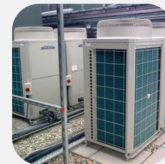
Variable refrigerant flow units
