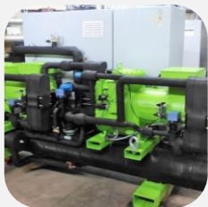
High temperature communal heat pumps
