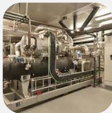
Standard temperature communal heat pumps
