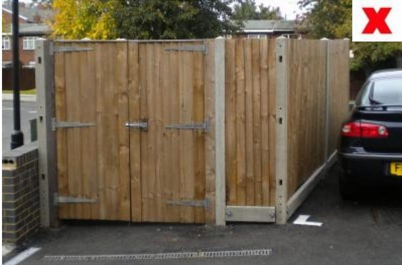
1. Inadequate screening. 2. Unacceptable - Timber frame vulnerable to impacts.
