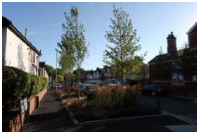
Figure 42 Example of SuDS incorporated in traffic calming measures and extended pavements (Source: SusDrain 29 )
