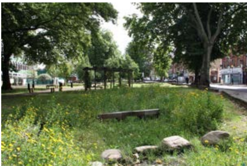
Figure 53 Example of detention basin within small green open space (Source: SusDrain 29 )
