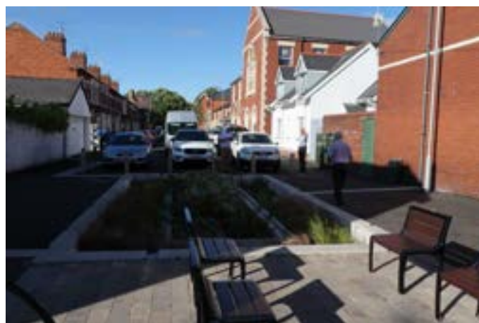
Figure 56 Example sunken raingardens providing flood storage in urban environments (Source: SusDrain 29 )
