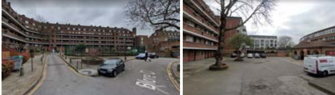
Figure 49 Paved areas in Blore Close and by Bilton House to be replaced with raingardens and permeable paving.
