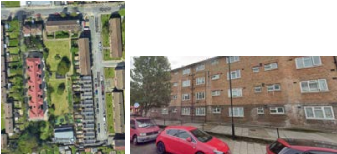
Figure 67 Astley House aerial view (opportunity for a detention basin) and from Gipsy Hill (opportunity for raingardens)
