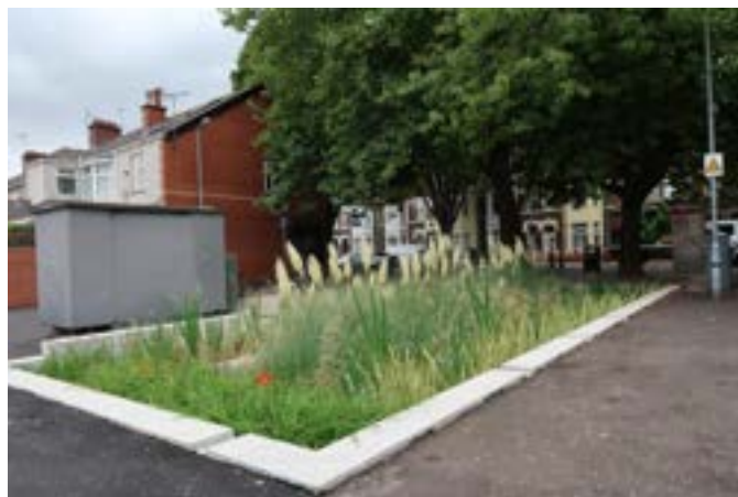
Figure 39 Example of green infrastructure providing flood storage in a pedestrian environment (Source: SusDrain 29 )
