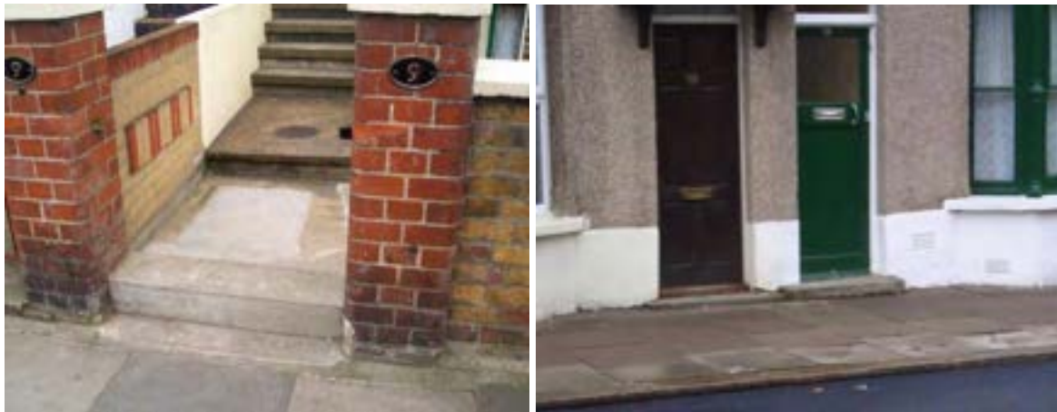
Figure 34 Example of raised property threshold (gate threshold on Dulwich Road and property threshold on Robson Road, LBL)
