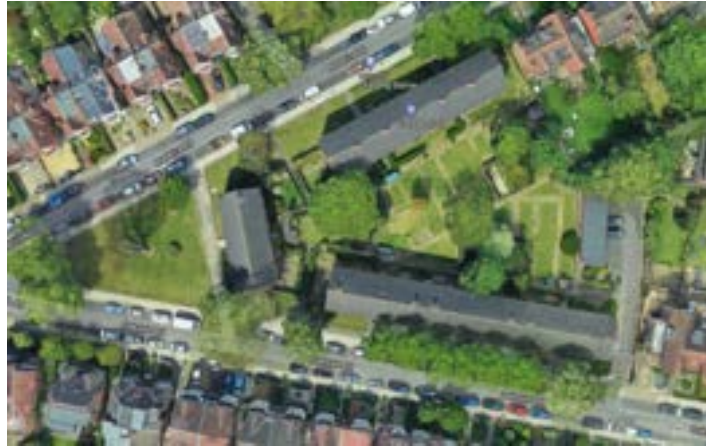
Figure 57 St Anselms Court Estate (opportunity for raingardens and tree pits)
