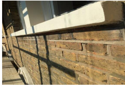
Example concrete repair and external decs, helibar below.
