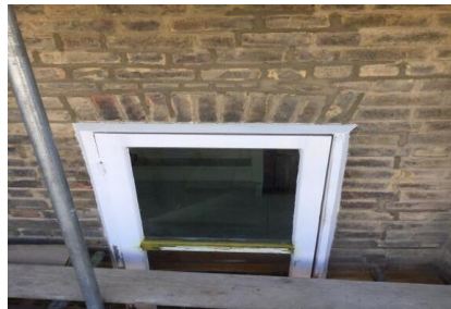
Window showing resin repair to cross piece. Repointing and helibar repair above.
