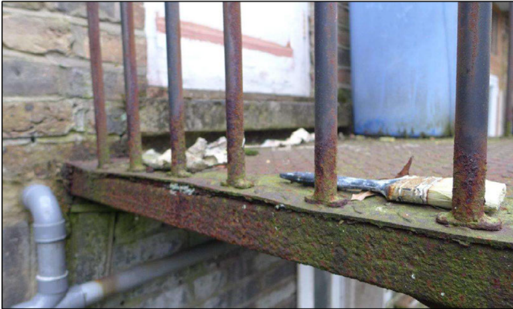
Photo 1: View of the top landing plate to the external staircase showing the general level of corrosion. Note the distortion to the plate caused by the expansion of the oxidising metal.
