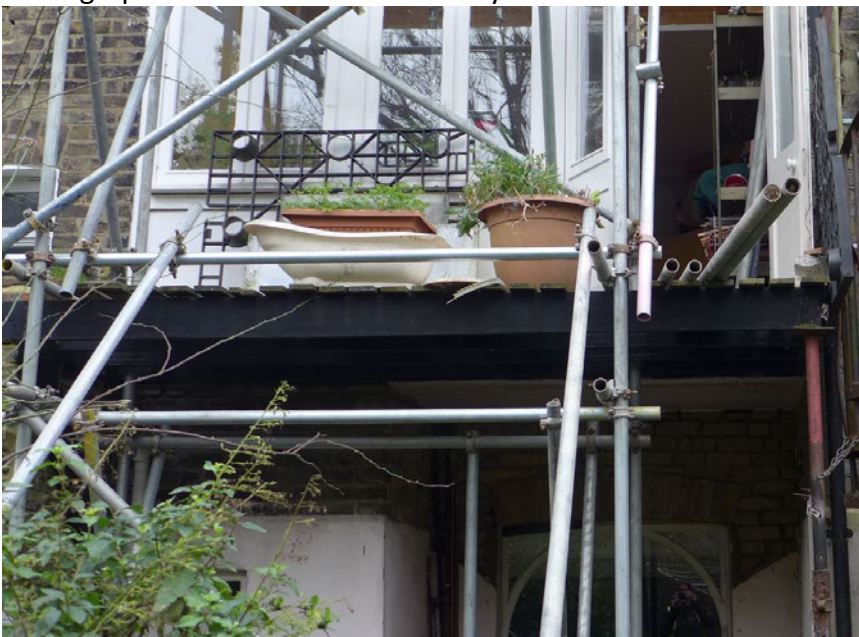
Photograph 2 – Unsafe timber balcony structure
