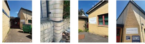
Existing Main Entrance
