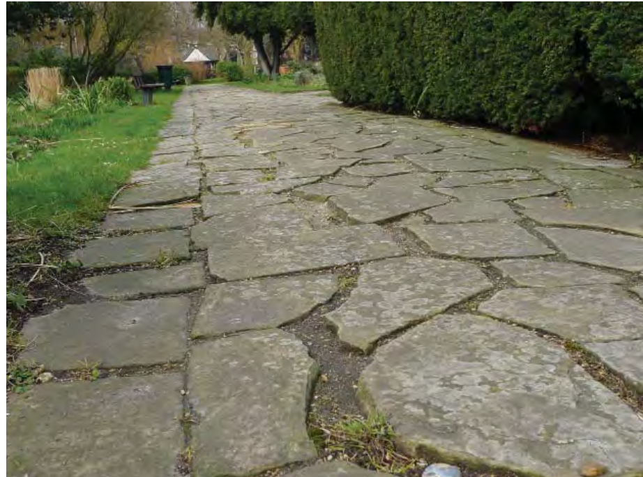
Figure 11 The Yorkstone crazy paving is in poor condition and uneven with open joints
