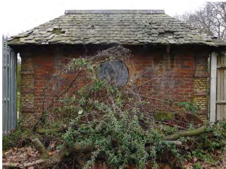
Figure 14 The pavilion roof requires urgent repairs to prevent further damage to the structure
