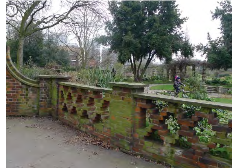
Figure 12 The original lattice brick wall forming the western boundary requires cleaning and repairs
