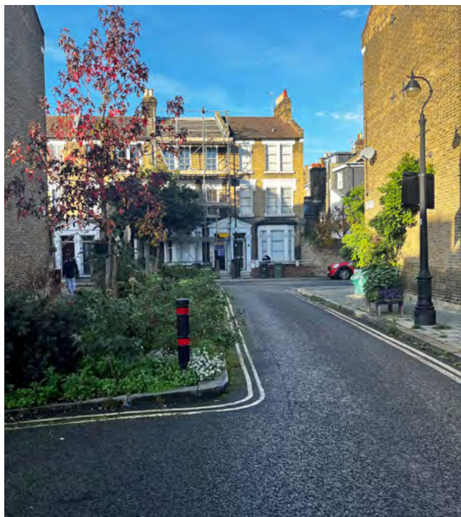
Tradescant Road, Oval. The pavement has been widened, calming traffic and providing space for plants which will soak up rainwater.
