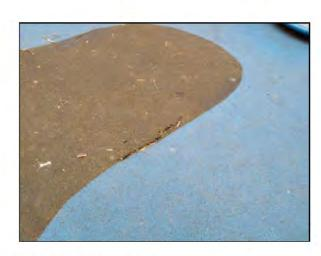
Finding: Action: The surface is lifting at the edges and creating trip points Repair perimeter of surfacing to remove trip points 1LM
