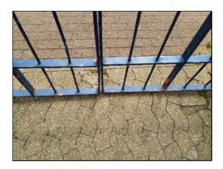
Finding: The gate has no drop bolt sleeves and/or drop bolts fitted
