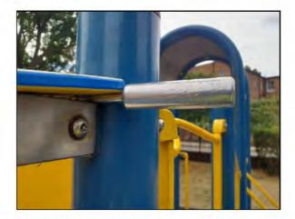
There is/are finger entrapment/s in the structure and the item fails to meet the requirements of BS EN 1176 Part 1 4.2.7.6 Entrapment of fingers Finding:
