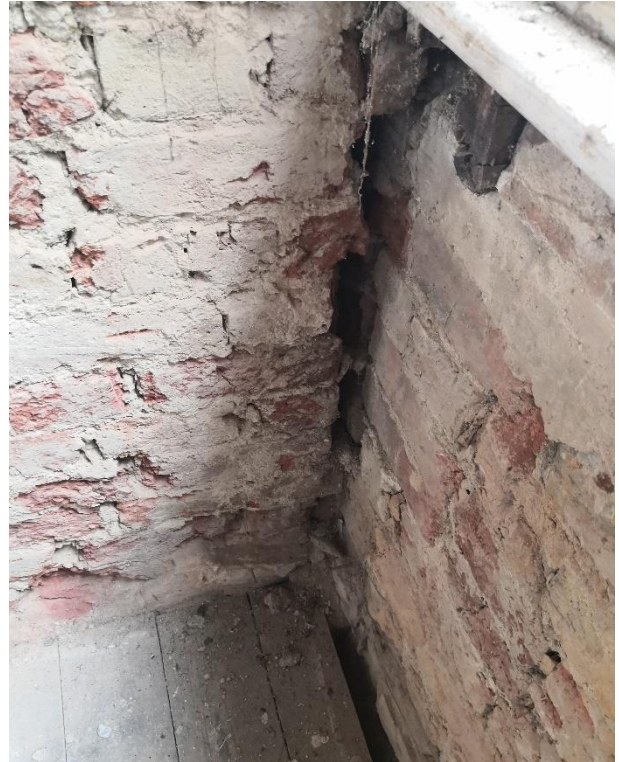
6.41 10-20mm wide gap in the corner of the stair landing between the rear elevation wall and internal wall with the large ground floor room (right)
