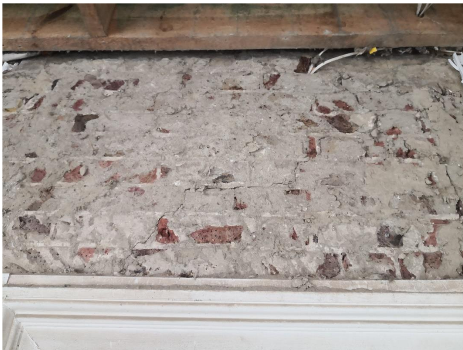
6.21 1-2mm wide cracks in the ground floor front left-hand room at the top left and right-hand corners of the door
