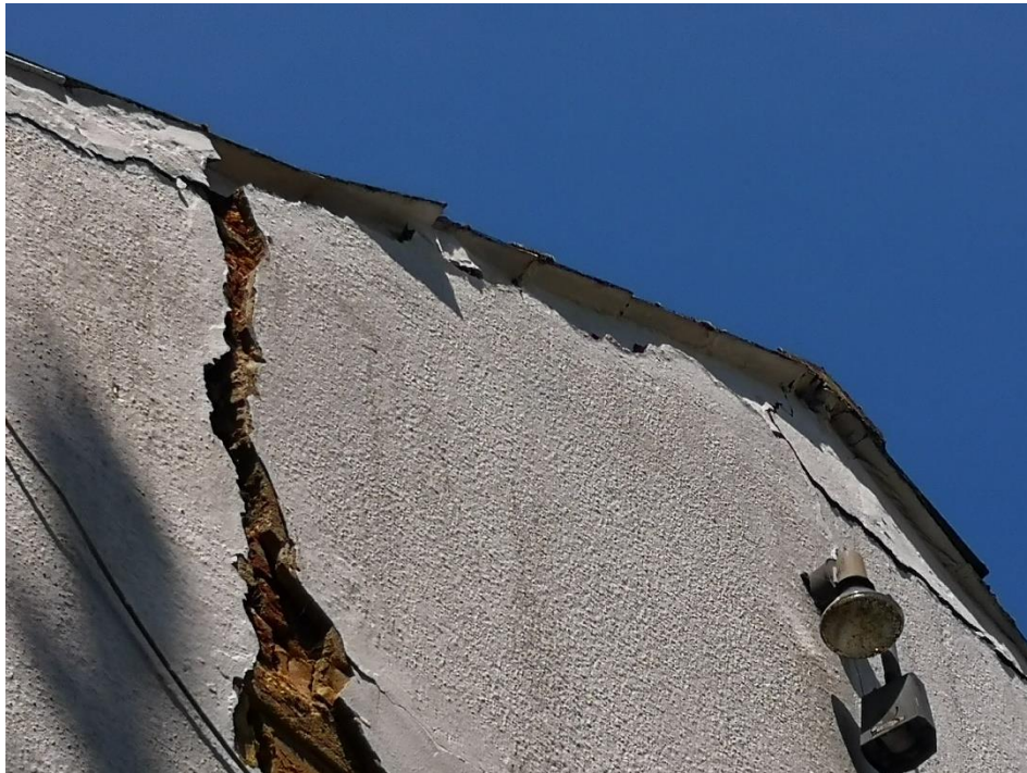
6.8 Significant cracks in the rear elevation at the top right and left-hand corners of the stair window. Note that the wall above the window appears to have moved outwards (right)
