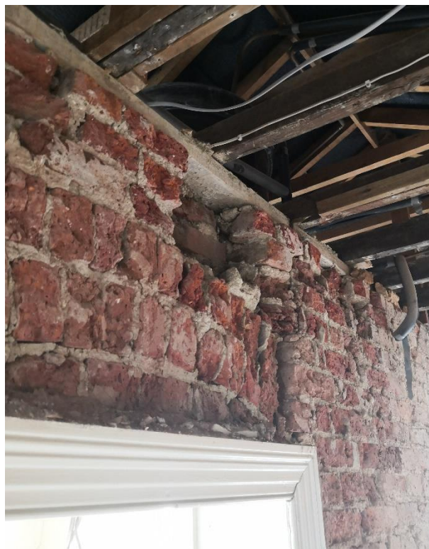
6.46 Example of area of masonry wall on the first-floor landing that has deteriorated.
