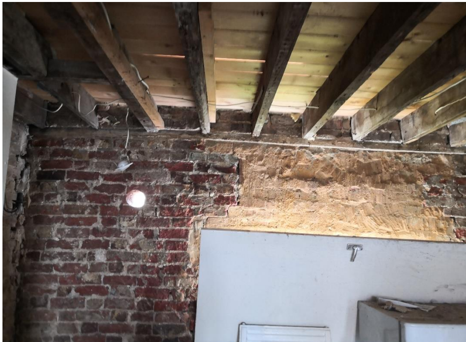
6.34 Rear elevation wall above the rear door opening in the ground floor right-hand room that is distorted
