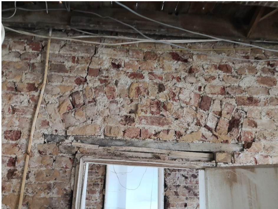
6.31 3-5mm wide crack in the ground floor right-hand room at the top left-hand corner of the front-most door to the hallway
