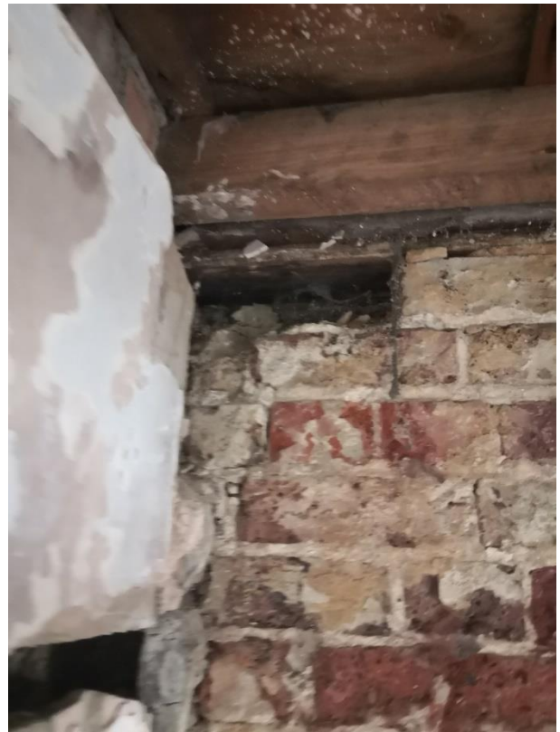
6.27 Hairline to 1mm wide crack in the ground floor back left-hand room in the right-hand window reveal (left)
