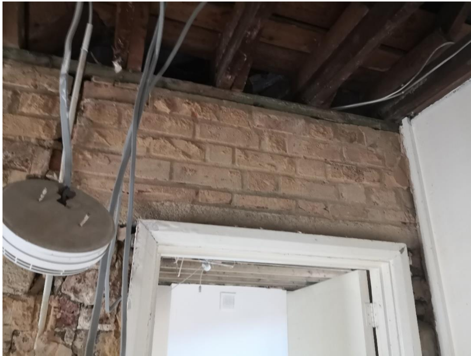
6.47 Area of newer masonry on the first-floor landing
