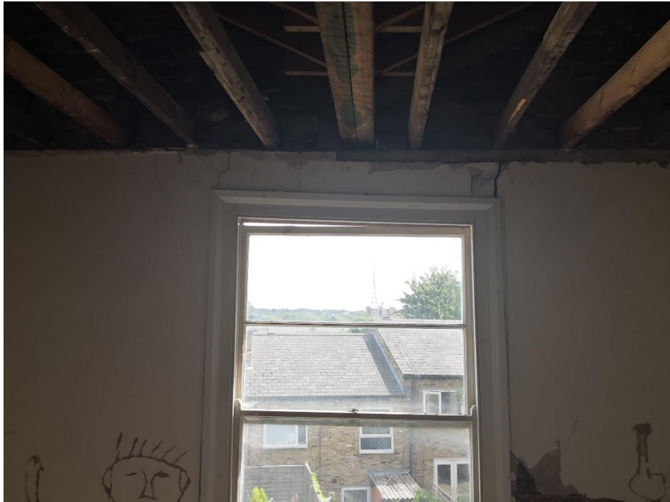
6.67 1-2mm wide crack in the first floor back right-hand room between the rear elevation and the party wall
