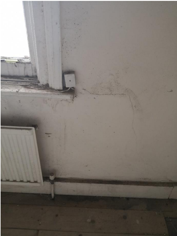
6.60 1-2mm wide crack in the first-floor front right-hand room at the bottom right-hand corner of the window (left)
