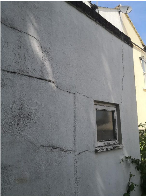
6.7 Numerous 1-3mm wide cracks in the rear elevation of the one storey section of the property (left)
