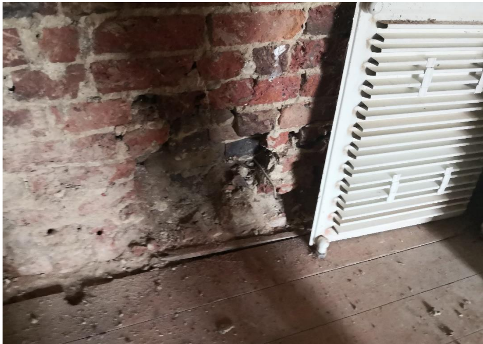
6.36 Area of masonry in the ground floor right hand room at low level on the right-hand side of the rear door opening that is missing (right)
