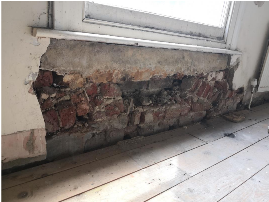
6.66 Area of deteriorated/missing masonry in the first floor back right-hand room below the window
