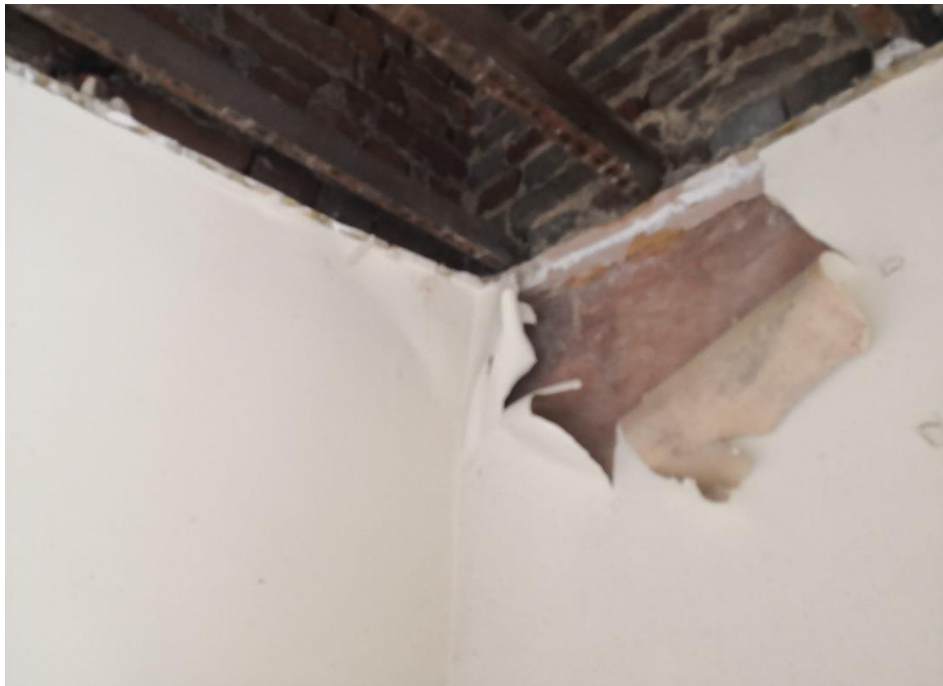
6.62 Evidence of water penetration on the wallpaper in the first-floor front right-hand room at high level of the front elevation wall
