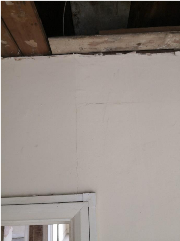
6.56 Hairline crack in the first floor back left-hand room at the top right-hand corner of the door (left)
