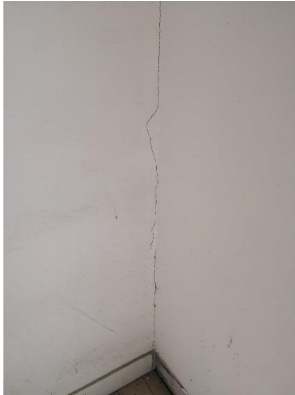
6.67 1-2mm wide crack in the first floor back right-hand room between the rear elevation and the party wall
