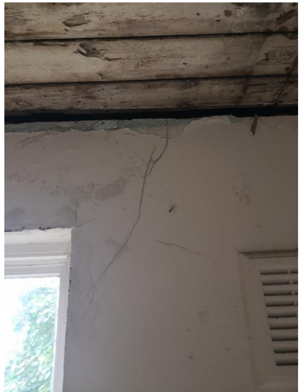
6.56 Hairline crack in the first floor back left-hand room at the top right-hand corner of the door (left)
