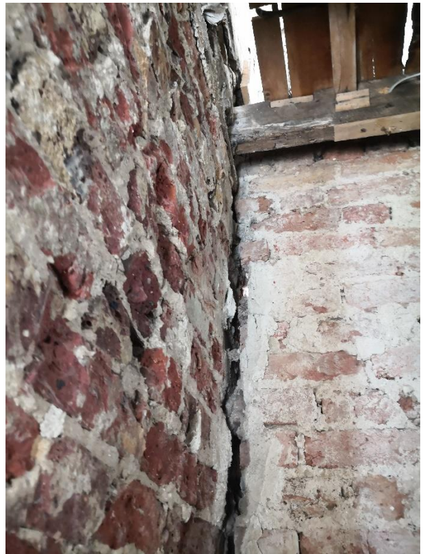
6.32 10-15mm wide crack in the ground floor right hand room at the top left-hand corner of the rear-most door to the hallway (left)
