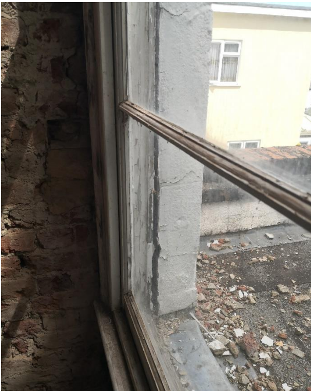
6.40 10-15mm wide gap around the stair window reveal (left)
