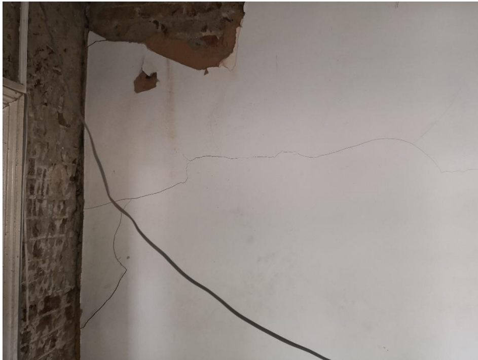
6.20 2-3mm wide crack in the ground floor front left-hand room in the internal wall with the ground floor back left-hand room
