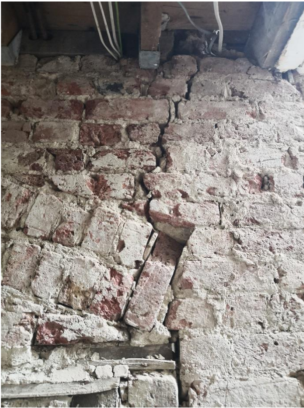
6.13 2-10mm wide crack in the ground floor hallway at the top right-hand corner of the rear-most door to the large room (left)
