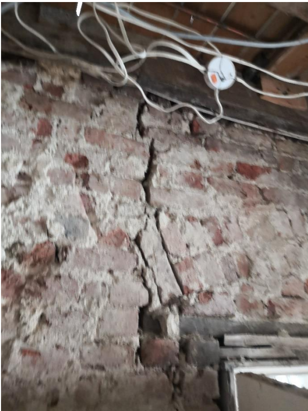
6.32 10-15mm wide crack in the ground floor right hand room at the top left-hand corner of the rear-most door to the hallway (left)
