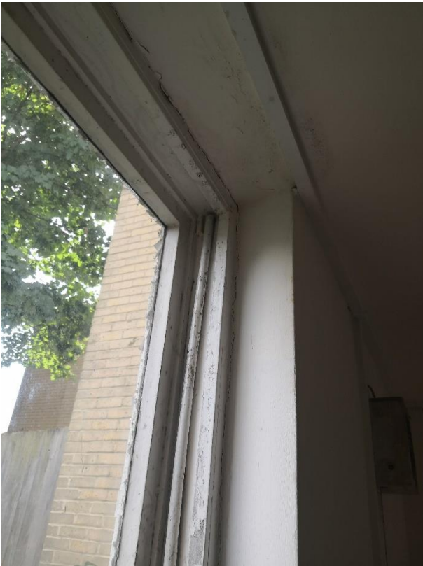
6.27 Hairline to 1mm wide crack in the ground floor back left-hand room in the right-hand window reveal (left)
