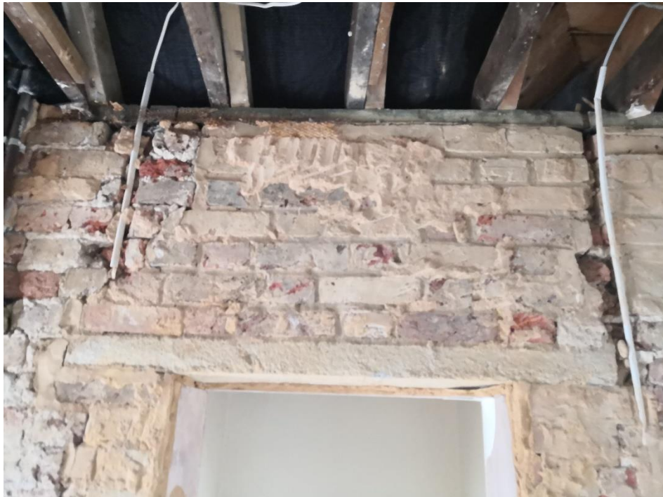
6.48 Another area of newer masonry on the first-floor landing
