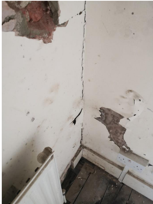
6.65 1-3mm wide crack in the first floor back right-hand room in the corner between internal wall with the stairs and the rear elevation wall
