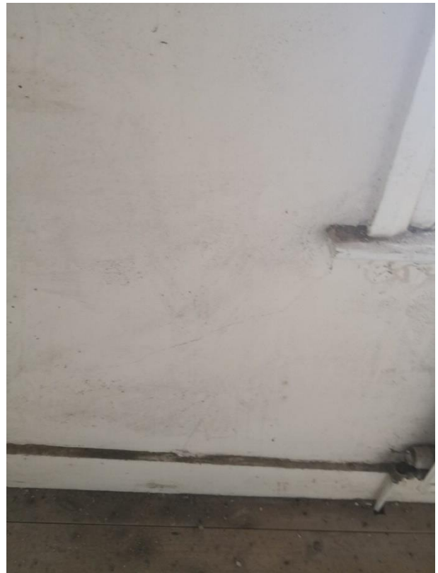
6.60 1-2mm wide crack in the first-floor front right-hand room at the bottom right-hand corner of the window (left)
