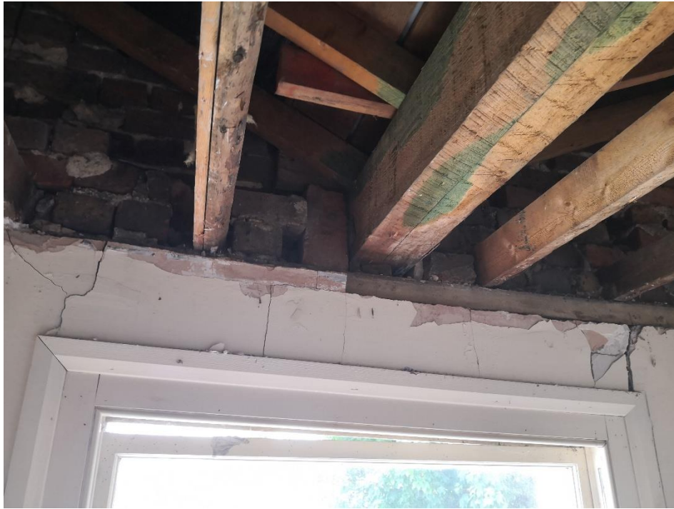
6.69 2-4mm wide crack in the first floor back right-hand room at the top left-hand corner of the window and 4-10mm wide crack at the top right-hand corner of the window
