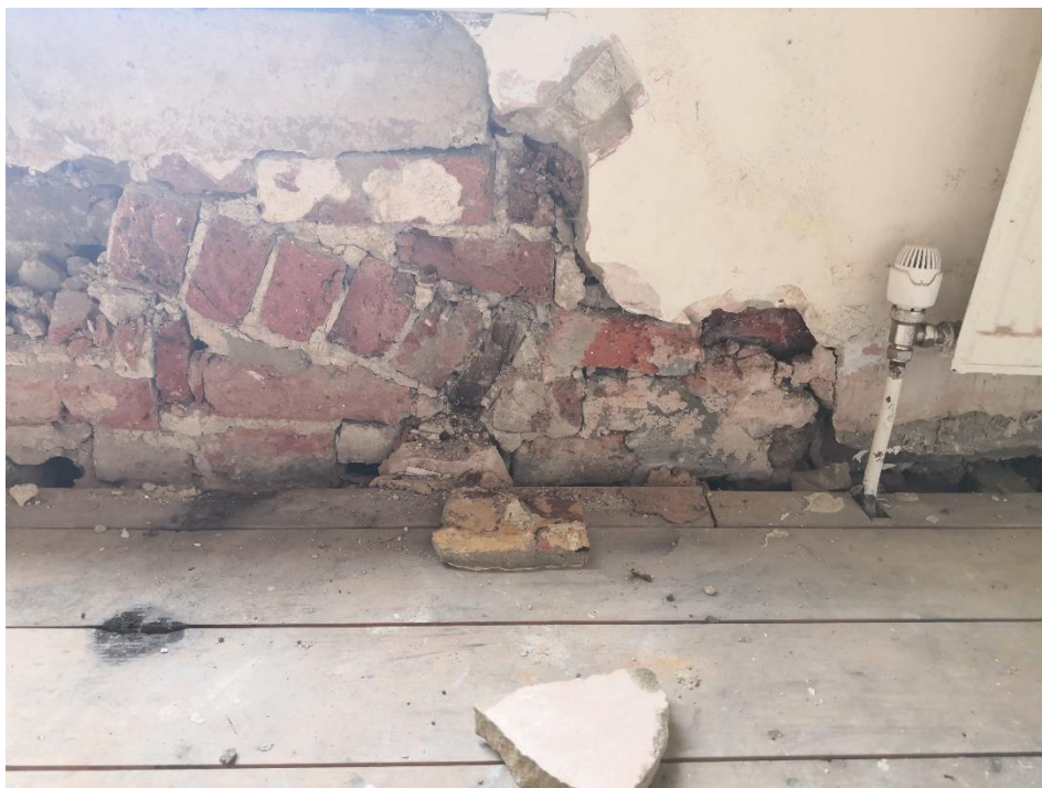
6.70 3-5mm wide crack in the first floor back right-hand room at the bottom right-hand corner of the window
