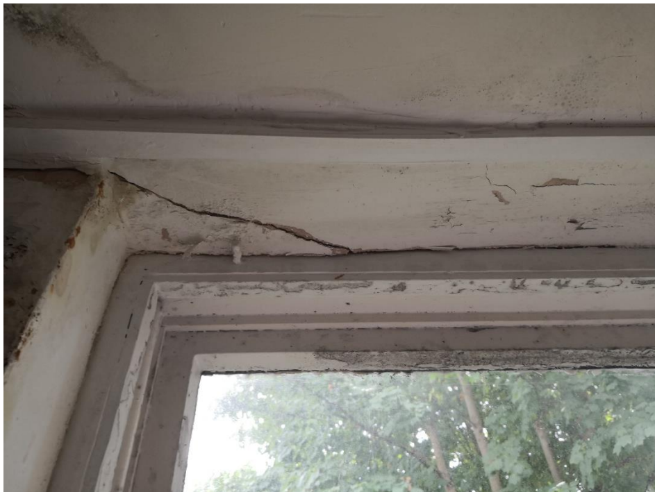
6.26 2-3mm wide crack in the ground floor back left-hand room in the top reveal of the left-hand window
