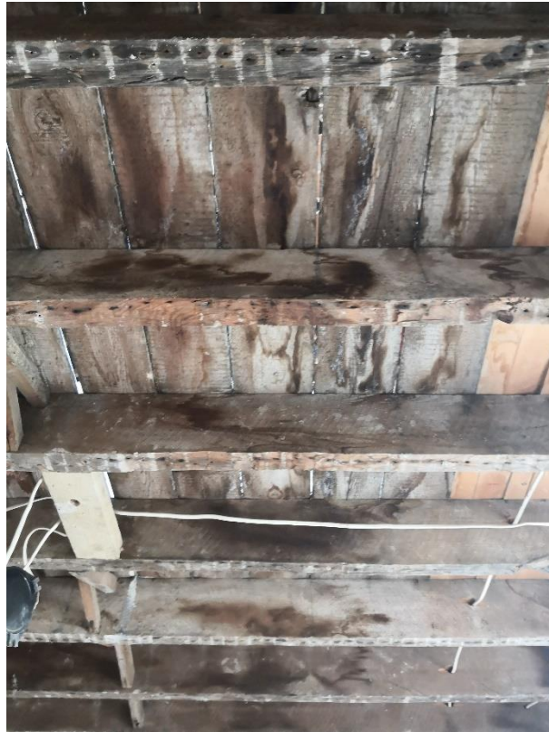
6.30 Efflorescent staining in the ground floor right-hand room on the underside of the first-floor floorboards
