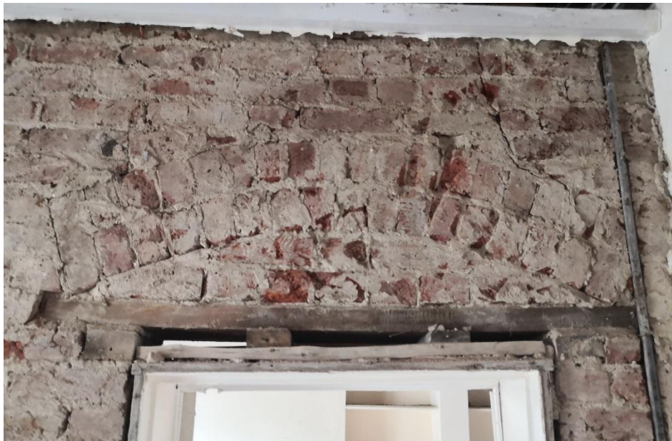
6.12 3-4mm wide crack in the ground floor hallway at the top right-hand corner of the front-most door to the large room
