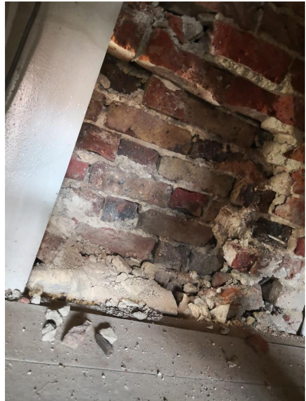
6.35 15-25mm wide crack in the ground floor right-hand room in the corner between the rear elevation and party wall (left)
