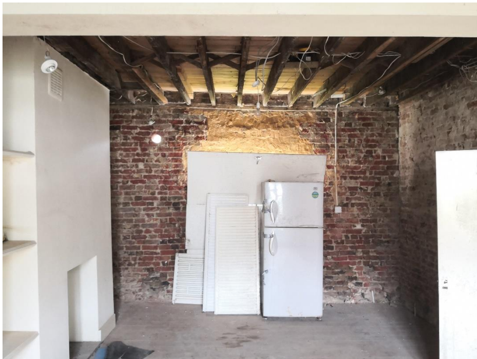
6.29 General view of rear door opening in the ground floor right-hand room. Note masonry above the door is distorted
