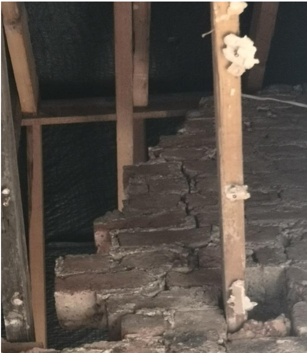
6.42 4-5mm wide crack in the stair area at high level on the internal wall with the back left room (left)
