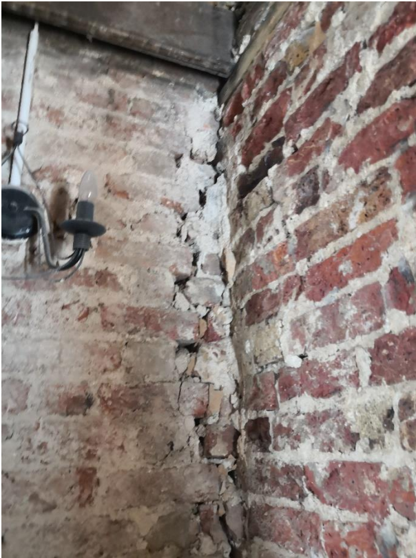
6.35 15-25mm wide crack in the ground floor right-hand room in the corner between the rear elevation and party wall (left)
