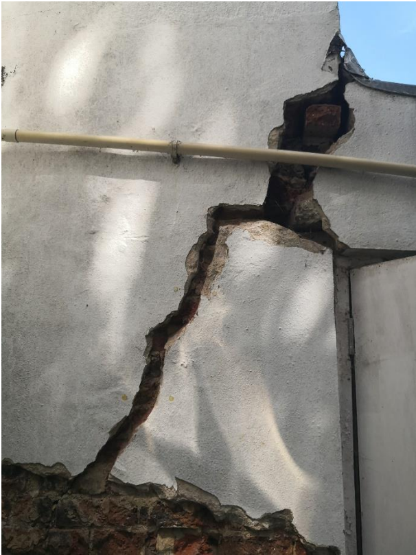
6.10 5-15mm wide crack on the left-hand side of the rear door on the side of the one storey section of the property (left)
