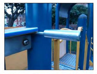
There is/are finger entrapment/s in the structure and the item fails to meet the requirements of BS EN 1176 Part 1 4.2.7.6 Entrapment of fingers Finding:
