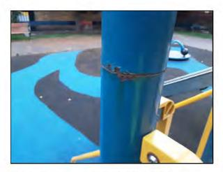
The paintwork on this item has been damaged or worn exposing the metal Finding:
