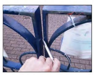
Finding: There are openings that are less than 12mm that could trap or crush fingers
