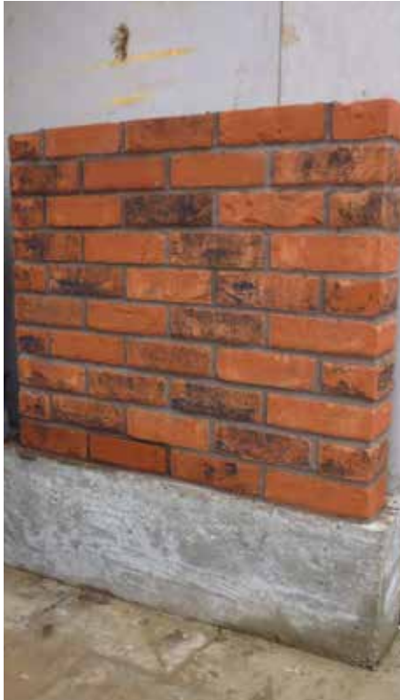
Sample panels constructed on site for approval
