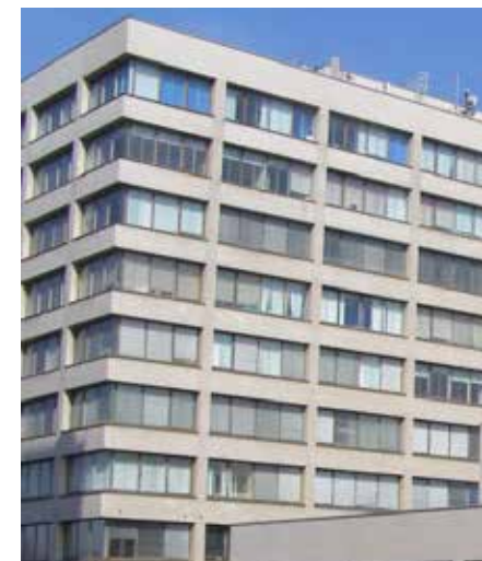
Cream tiles at St Thomas' Hospital
