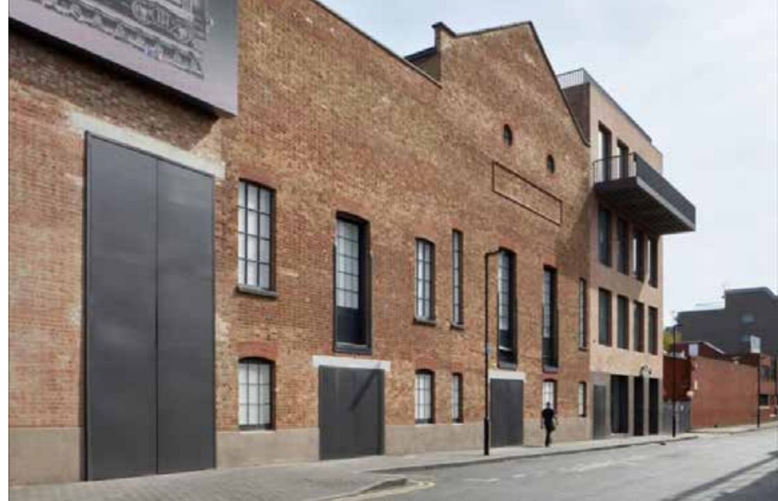
Newport Street Gallery by architects Caruso St. John - winner of Stirling Prize 2016
