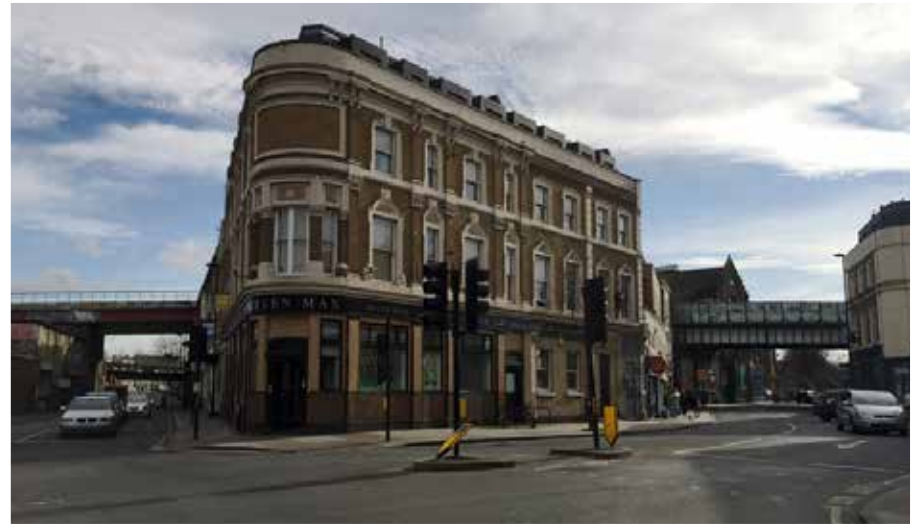
Prominent railway engineering
