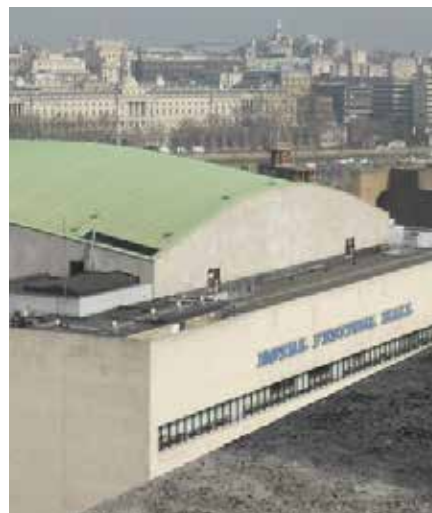
Portland Stone buildings
