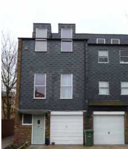
Mid-20th Century terrace, Myatt's Field South Estate
