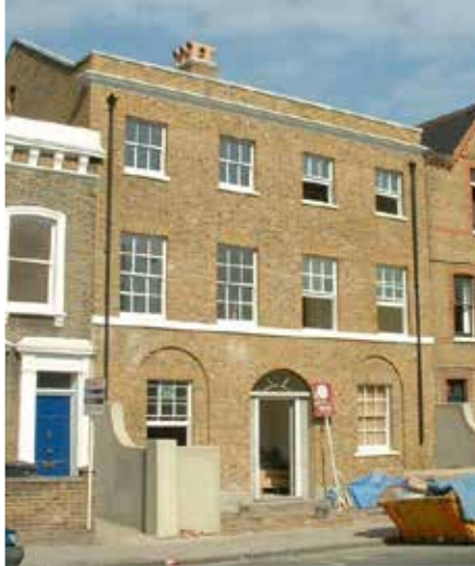
Georgian House, Larkhall Lane
