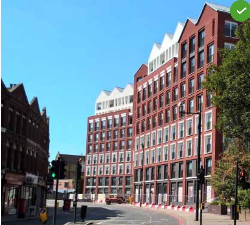
Contemporary design reinforces local character
