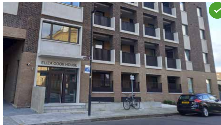
Convenient entrance with steps and level access
