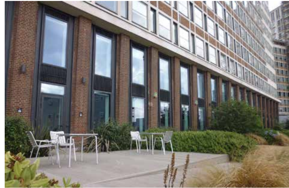
Office with outside amenity space
