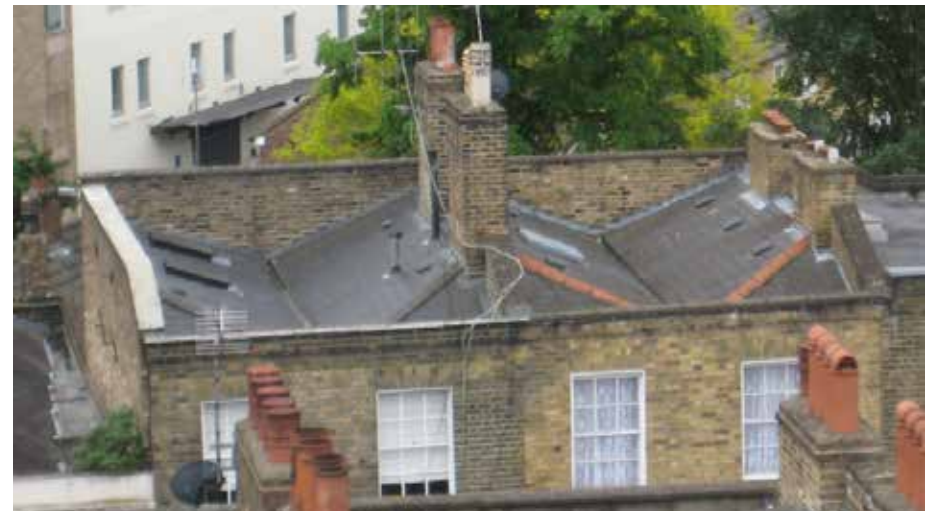
Earlier variation on a London roof c1810s when form was used to hide cheaper roofing materials such as pan tiles
