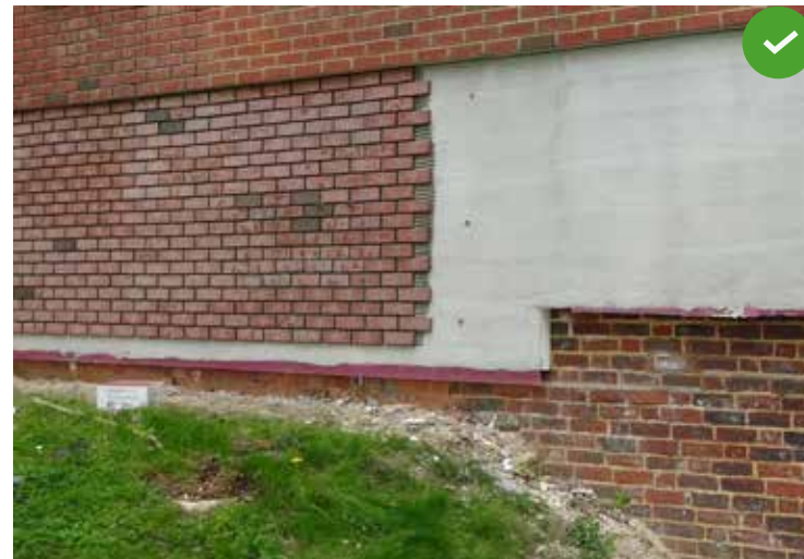
Brick slips over the insulation layer
