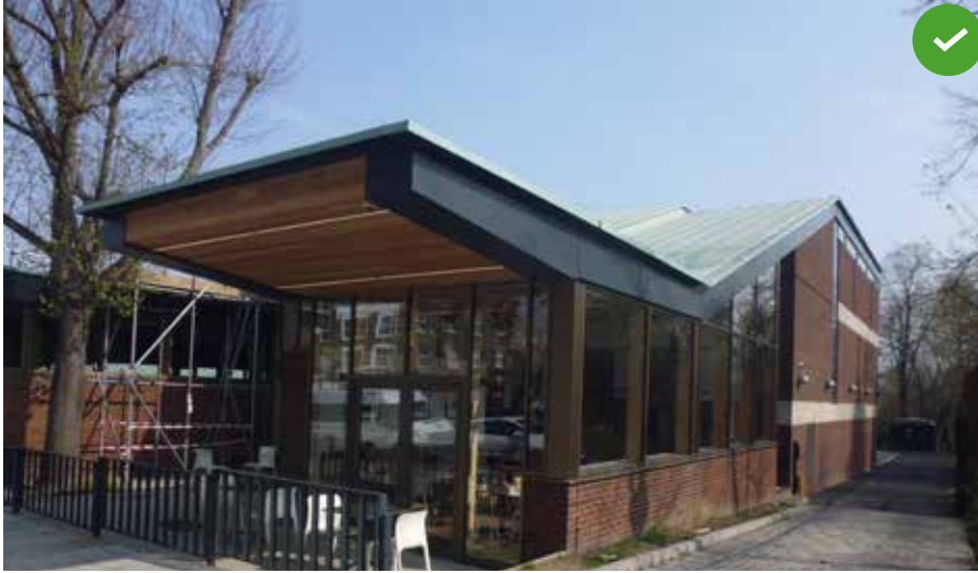
Sympathetic materials used on library extension
