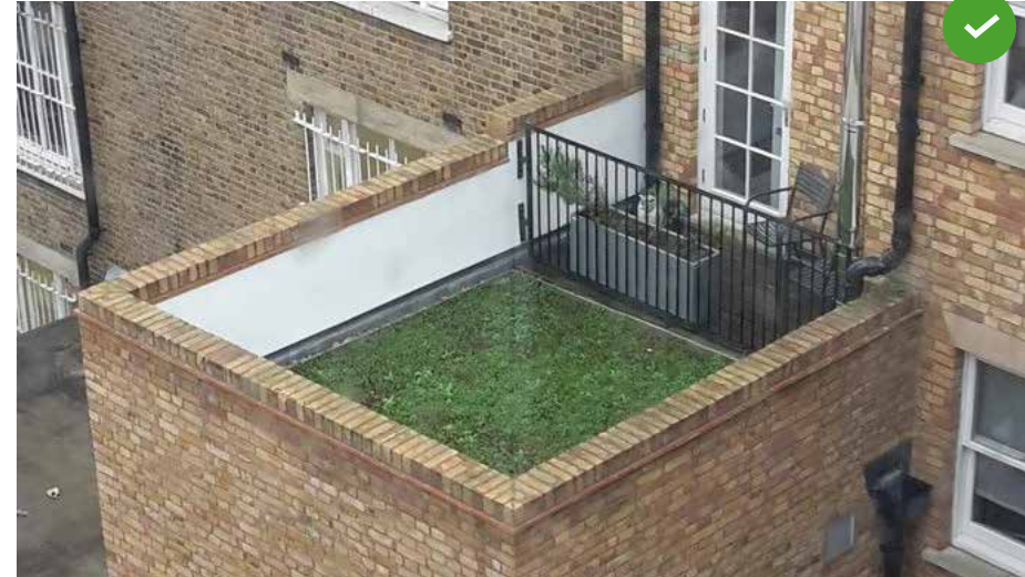
Green roof on extension
