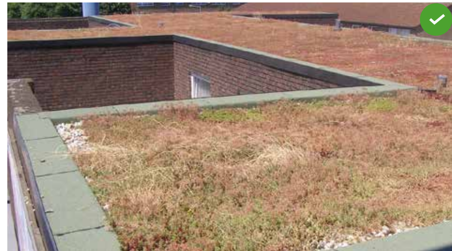
Retrofit green roof on Ethelred Estate
