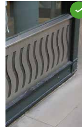
Vents in stallriser
