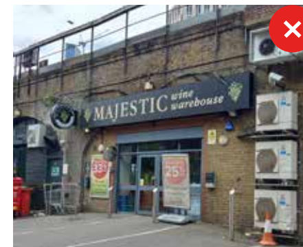
Arch features screened by signage and plant
