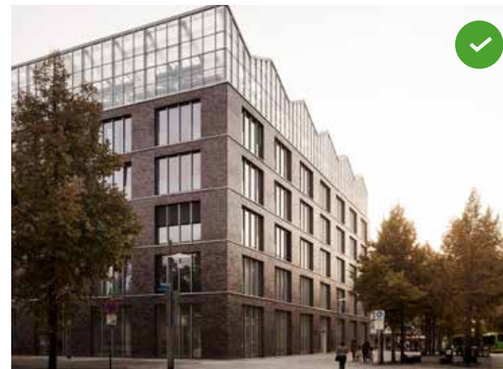
Integrated rooftop plant, here enclosed within a greenhouse
