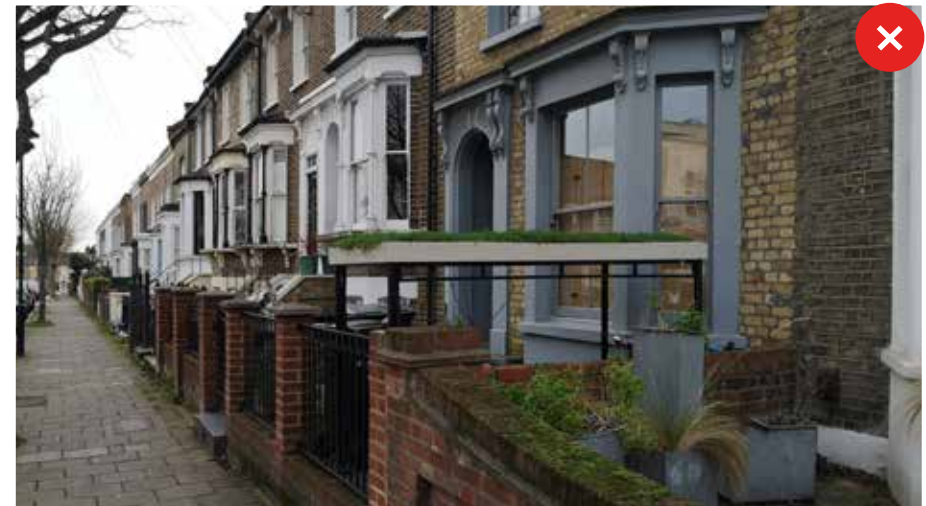
To protect visual amenity structures should be low
