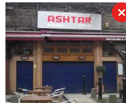
Poorly integrated awning and signage
