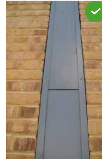
Gas pipes integrated
