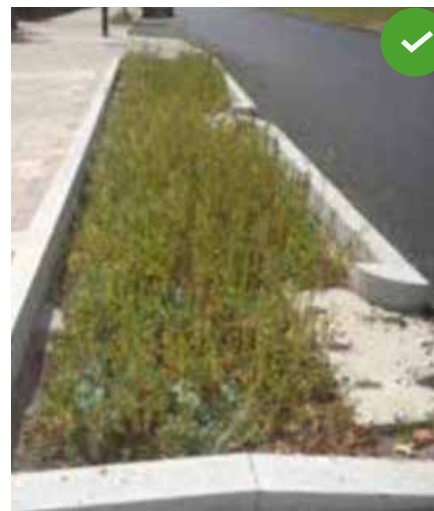
De-paving with kerb inlet in Streatham, Lambeth (After)
