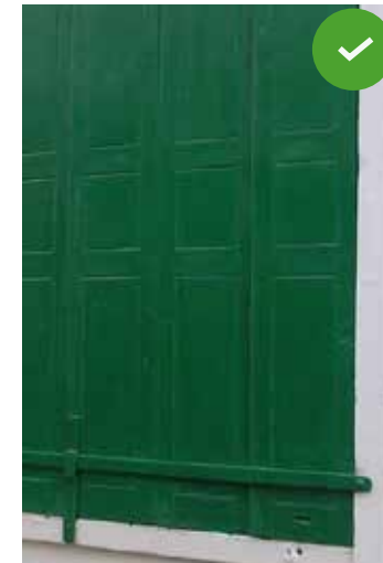
Traditional timber shutter
