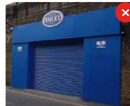
Arched profile covered
