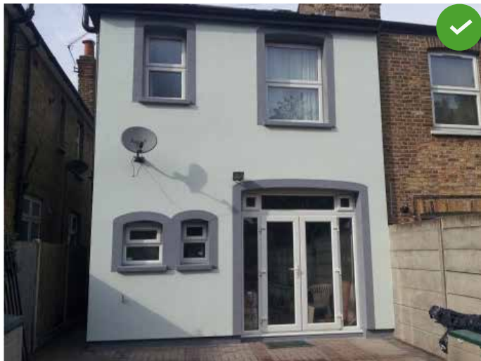
After - Render over insulation layer
