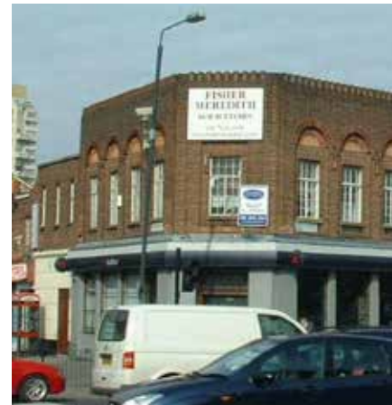
Before additional storey
