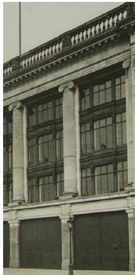
The loss of historic glazing in this façade retention has harmed the integrity of the retained façade.
