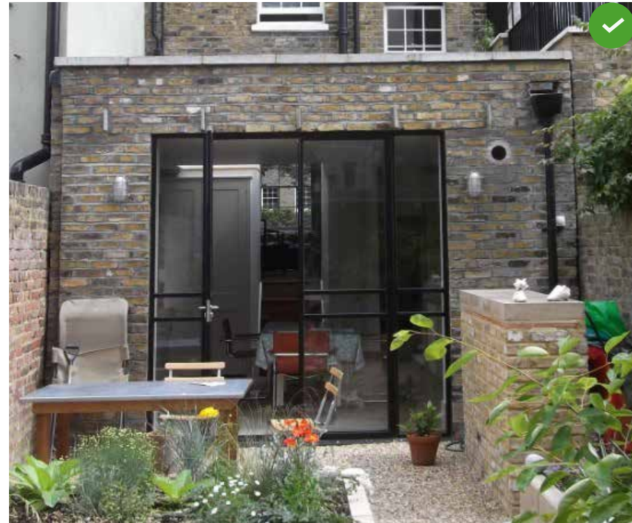
A full width extension on a modest terraced property
