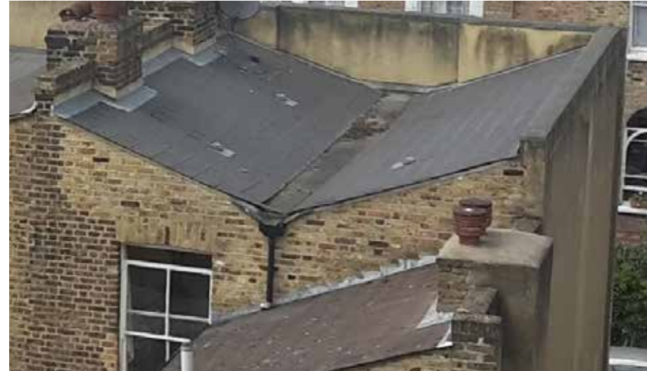
Typical London roof c1870s
