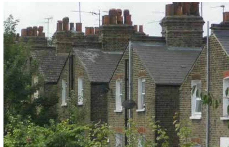
Rear return roofscape can contribute to local distinctiveness
