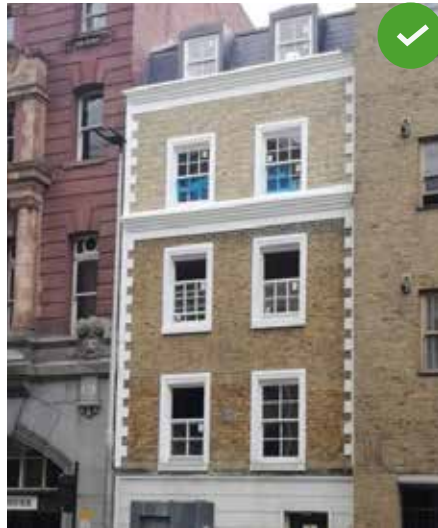
After to additional storeys
