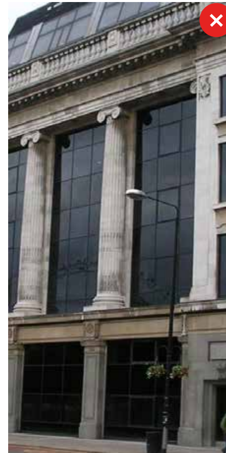
The loss of historic glazing in this façade retention has harmed the integrity of the retained façade.
