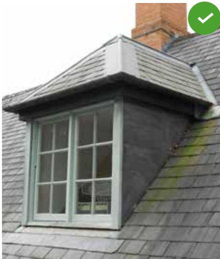
Neat construction detailing
