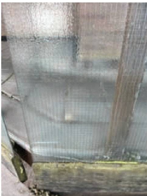
Wood - Poor Beads - internal - Generally poor.
