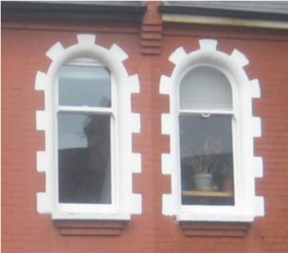
Figure 13 - Poor matches to the original windows, such as the example on the left, harm the special interest of the conservation area.
