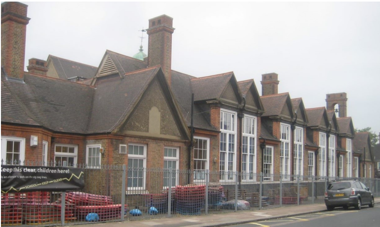
Figure - 3 The impressive frontage of Telferscot School to Radbourne Road
