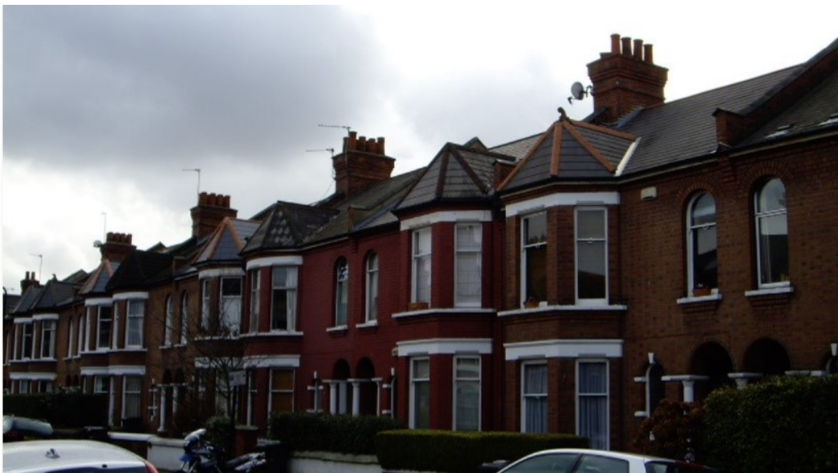
Figure 1 - Glenfield Road—canted bays groups in pairs.
