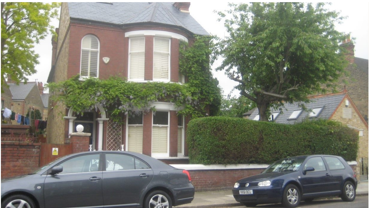
Figure - 2 No. 77 Midmoor Road is detached
