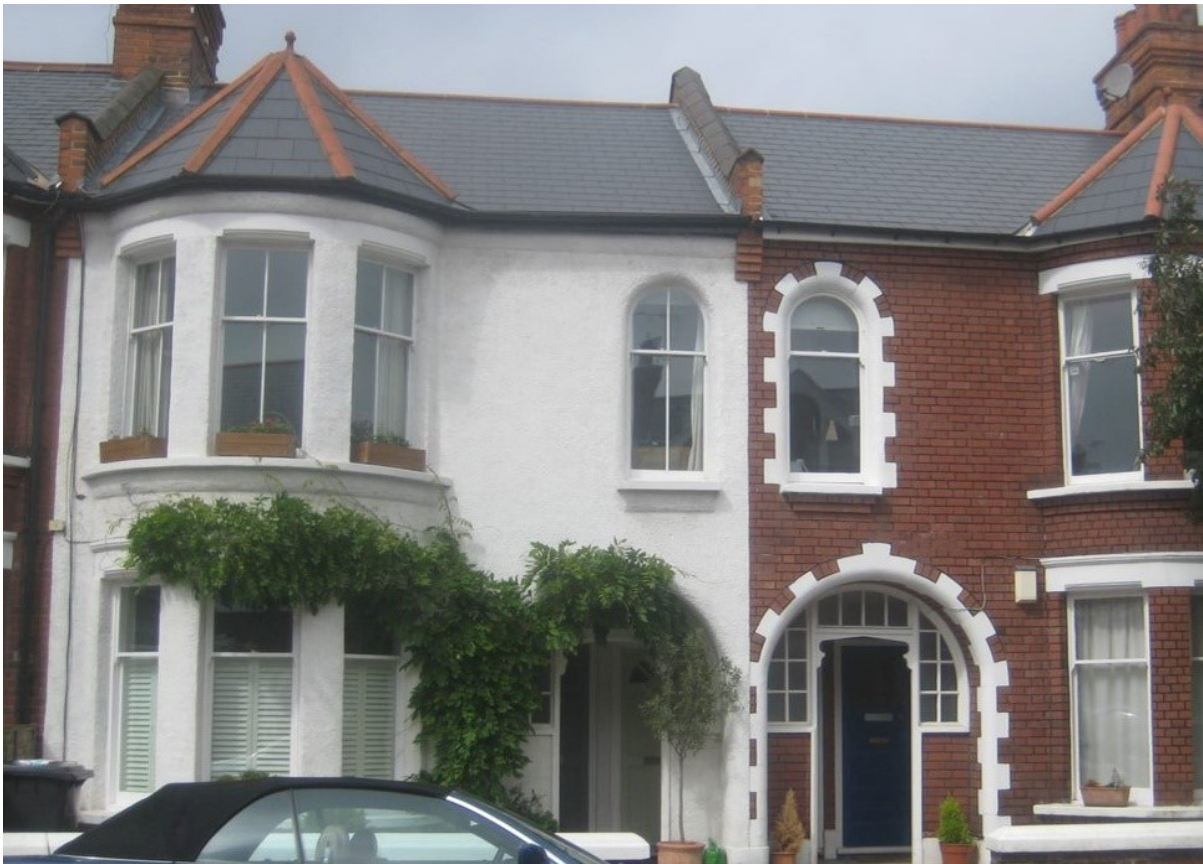
Figure 11 - The rendering of this properties harms their architectural integrity and the character and appearance of the conservation area.
