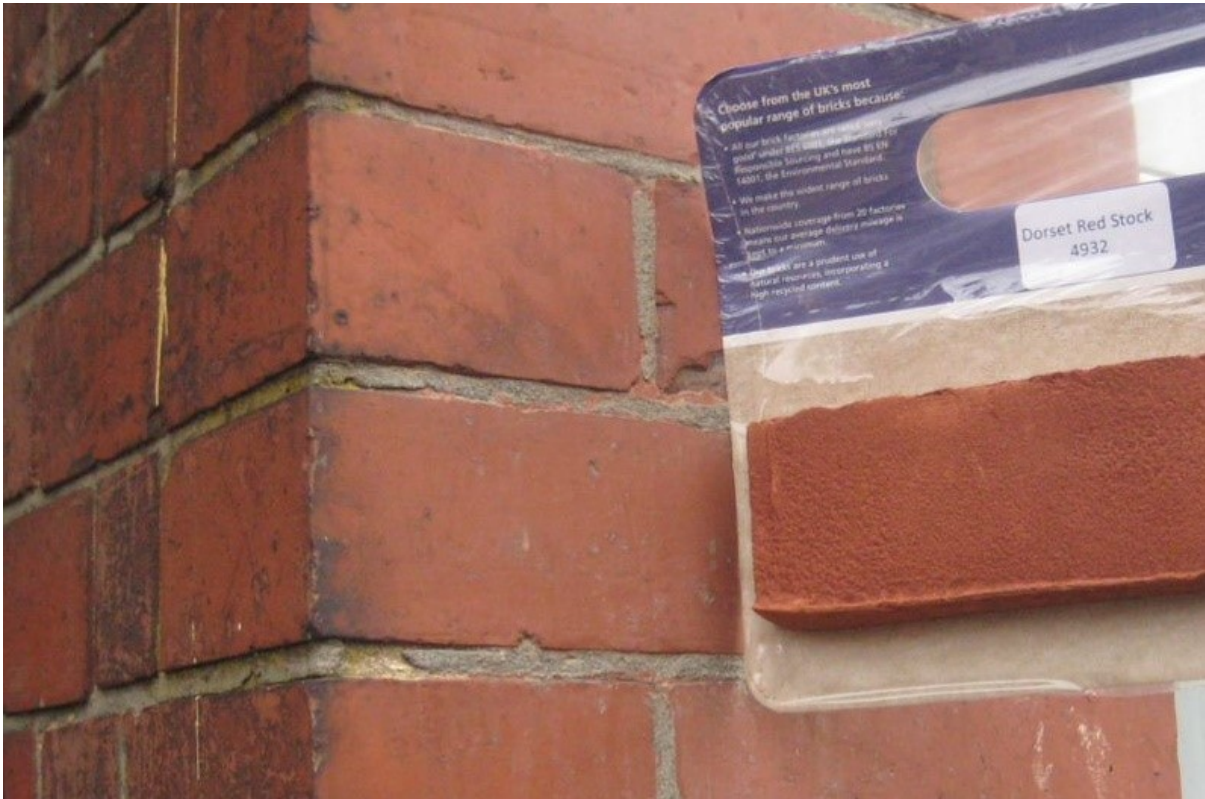
Figure 10 - Replacement bricks must be a close match to the originals.
