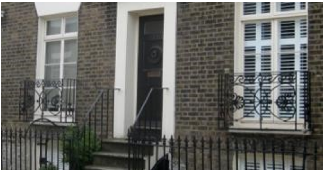
Traditional casements with ornamental balconettes—St Mary’s Gardens
