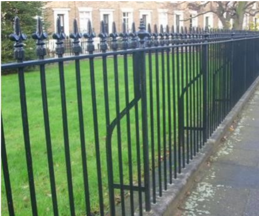
Traditional railings on Walcot Square—note the standards with braces and larger finials.
