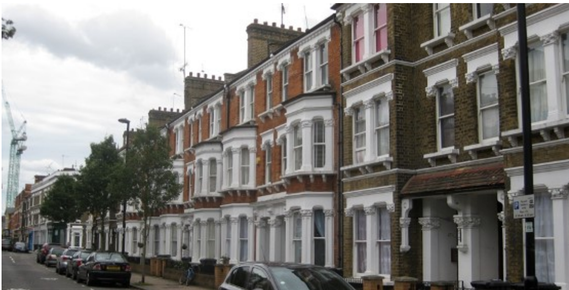
The ornate late Victorian terraced houses of Brook Drive.
