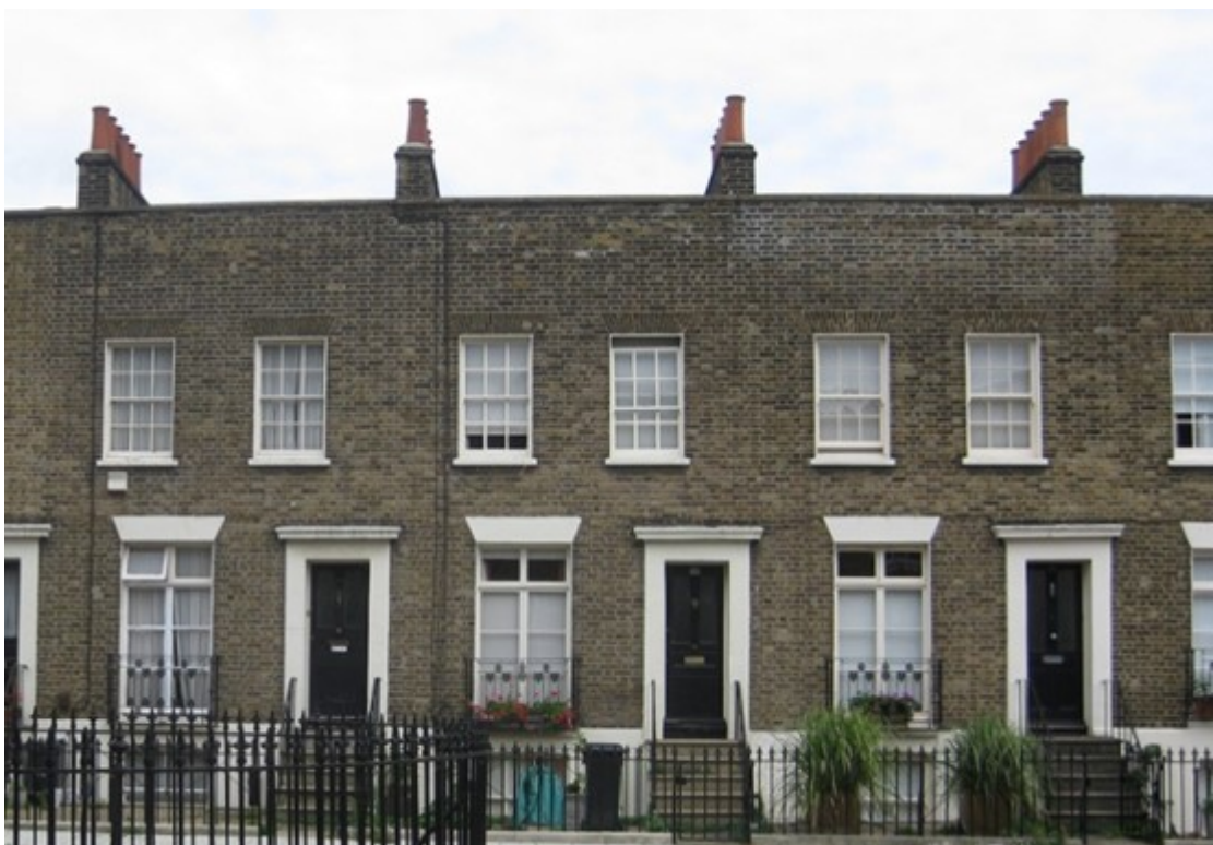
Historic houses with parapets do not have rainwater downpipes on their facades.
