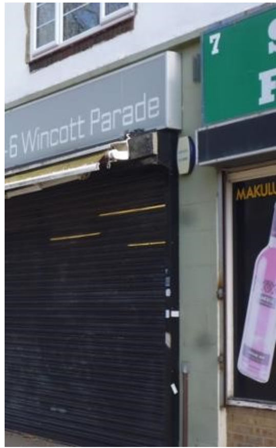
Unsympathetic signage and shutters
