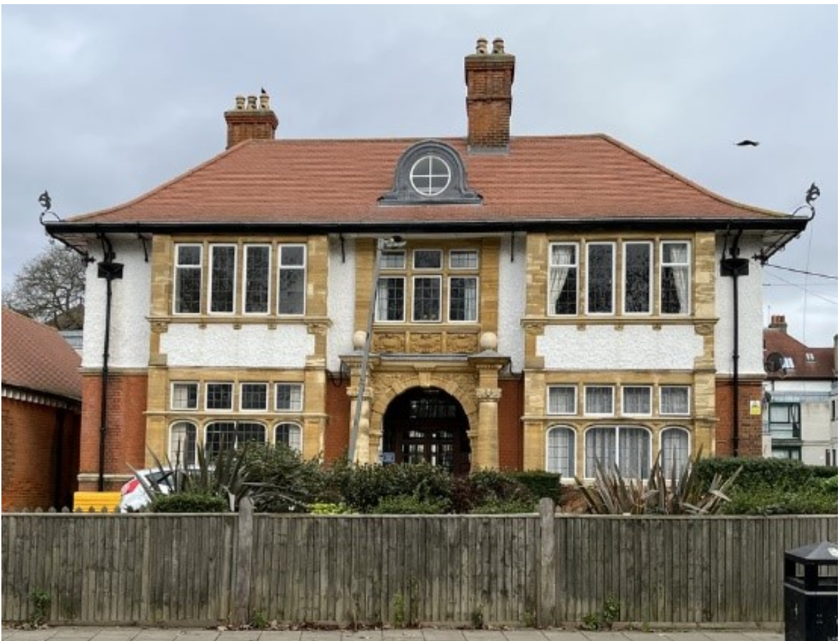
No. 23 Garrads Road has a symmetrical façade off-set with asymmetrical chimneys
