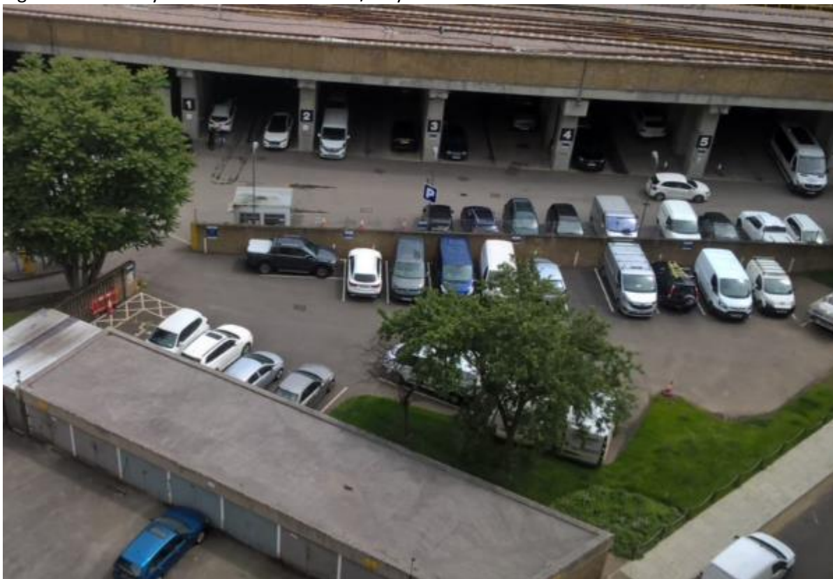
Figure 13 - Railway Viaduct at rear of Canterbury House
