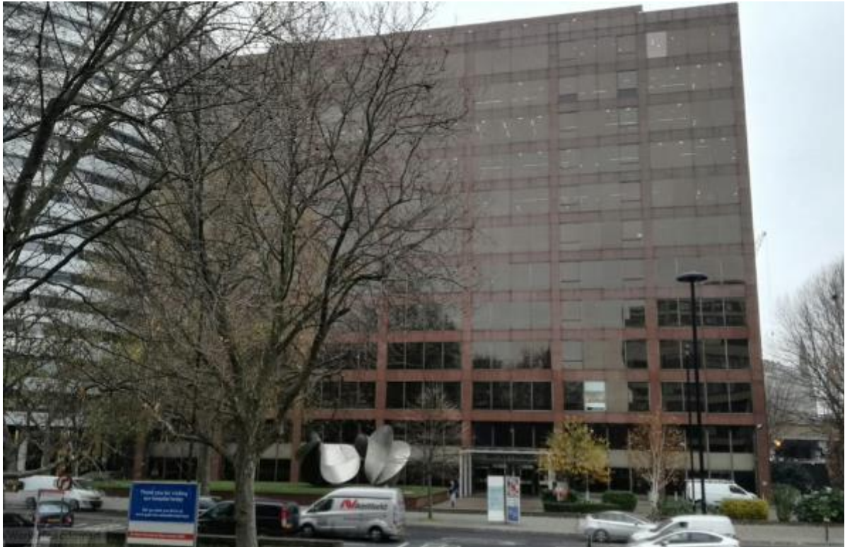
Figure 8 – Beckett House, Lambeth Palace Road
