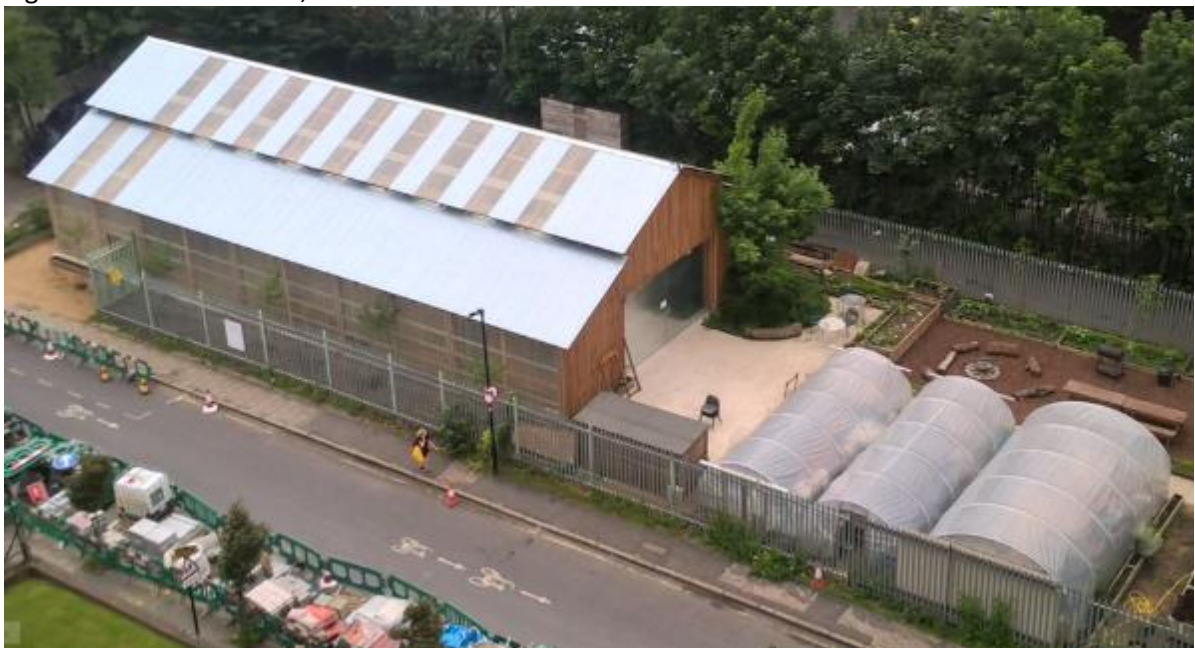
Figure 9 - Meanwhile use farm barn fronting Royal Street
