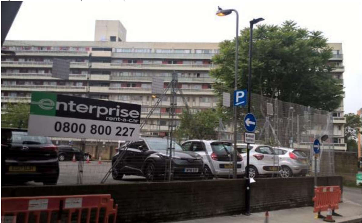
Figure 11 - Rear of Canterbury House viewed from Upper Marsh
