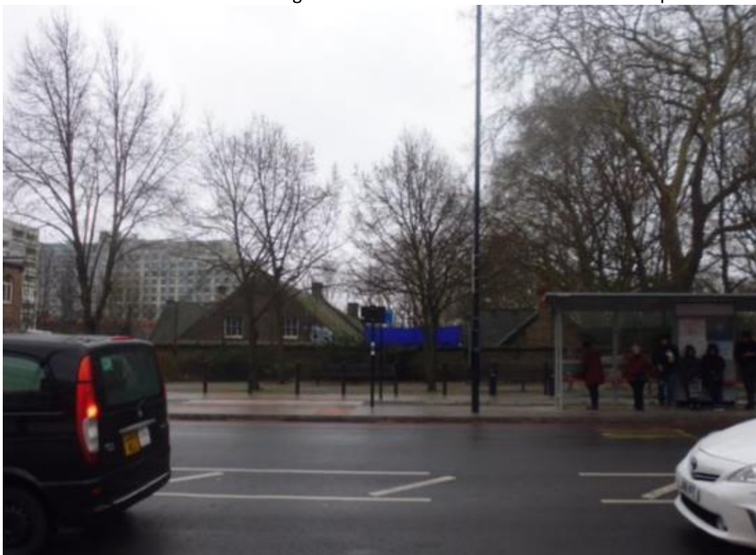
Figure 7 – former Christchurch School from Lambeth Palace Road
