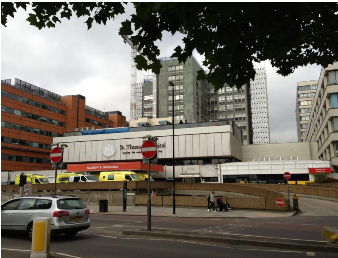
Figure 5 - A&E building viewed in context with East Wing (to rear) and Evelina Hospital (to left)
