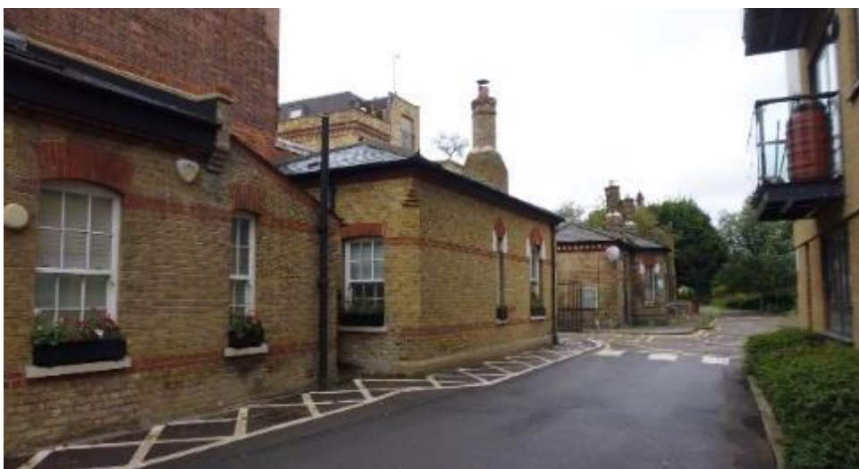
Figure 14 - Main entrance to workhouse and hospital site is between locally listed gate lodges
