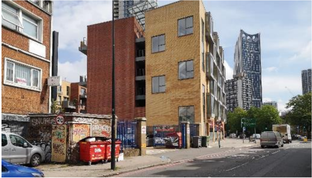
Figure 5 - The eastern end of the site frontage to Kennington Lane showing neighbouring property and the cramped and cluttered frontage treatment of the site.
