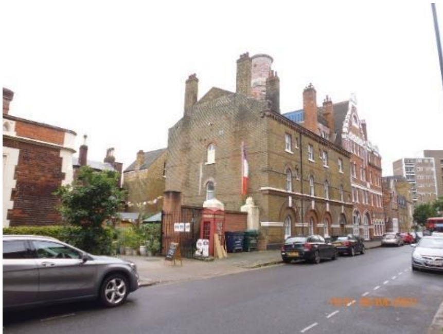
Figure 13 - Former Fire-station, Renfrew Road and the telephone kiosk (both grade II)
