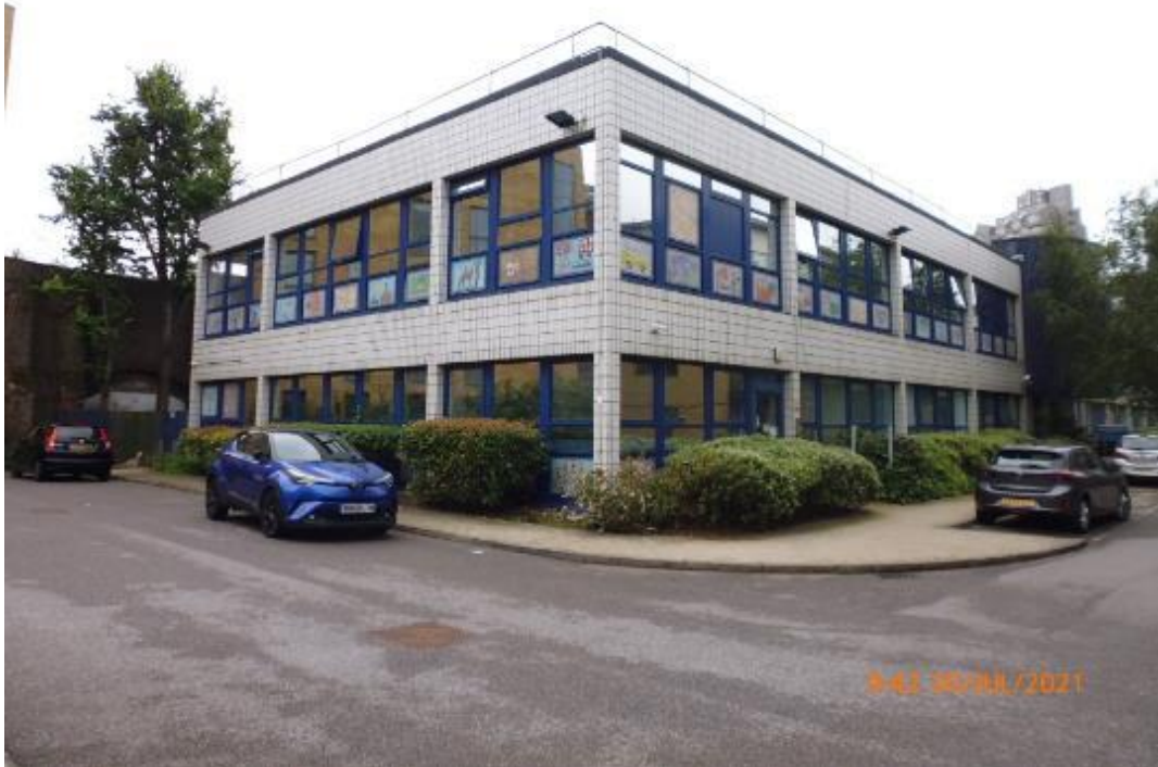
Figure 7 - Wooden Spoon House, Dugard Way.
