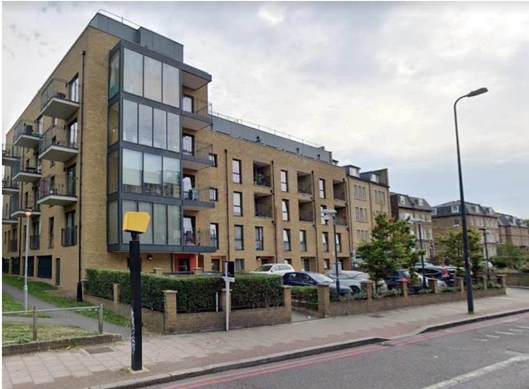
Figure 9 - No. 235 – 243 Brixton Road 'after'
