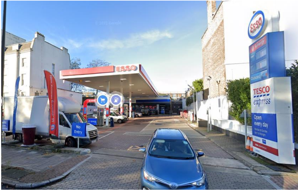
Figure 4 - The petrol filling station has a very poor effect on the conservation area.
