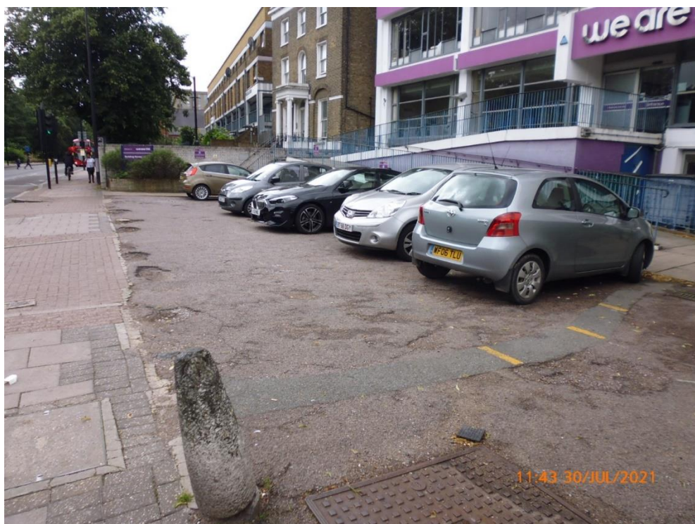
Figure 10 – On Brixton Road vehicle crossovers compromise pedestrian safety
