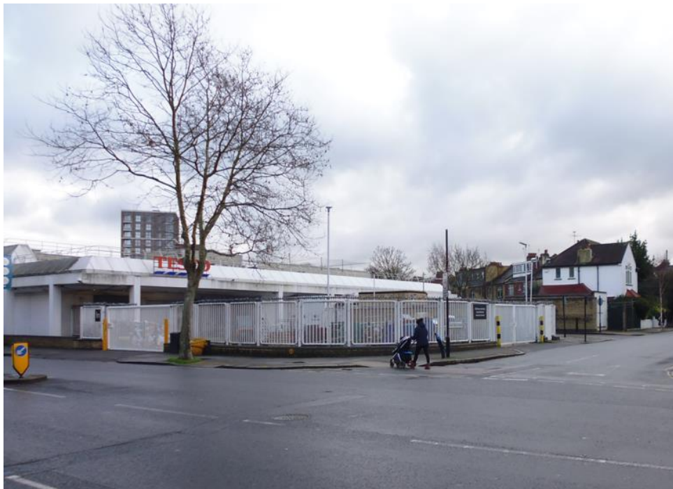
Figure 5 – Acre Lane – Tesco store service yard at corner of Baytree Road.
