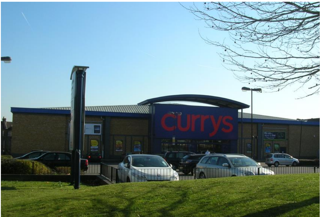
Figure 5 – Currys unit, Effra Road
