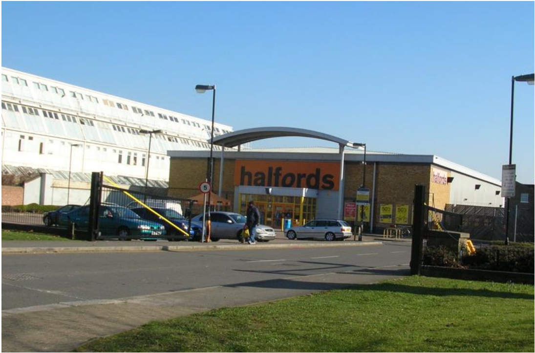
Figure 4 – Halford’s unit, Effra Road
