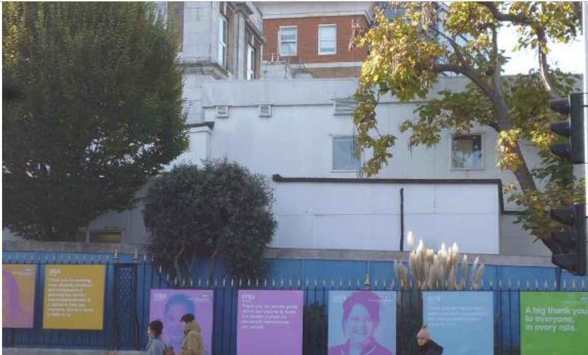
Figure 4 – Prefabricated buildings occupy prominent location on the Denmark Hill frontage
