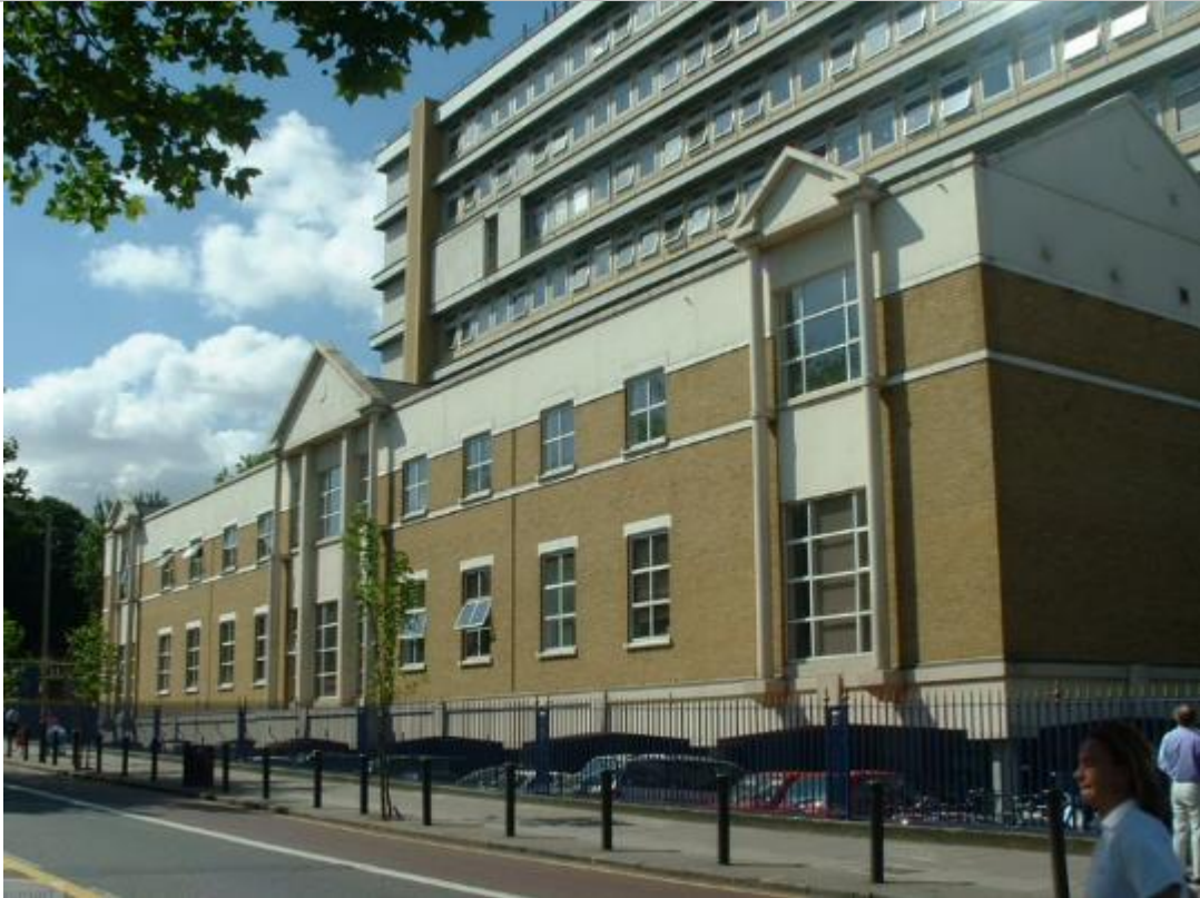
Figure 3 – The architectural quality across the campus lacks coherence
