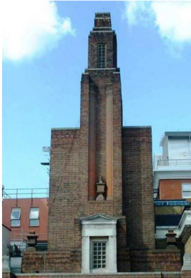
Figure 9 - The frontage block of the Guthrie Wing (local list) is retained.
