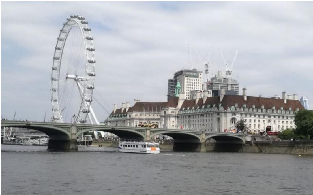
Figures 10 and 11 – The County Hall makes a High contribution to the setting of the WWHS.
