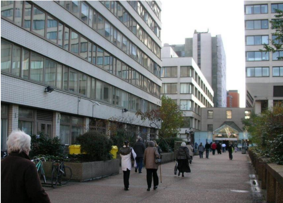
Figure 36 - Existing walkway with Western elevation of Gassiot House on left side.
