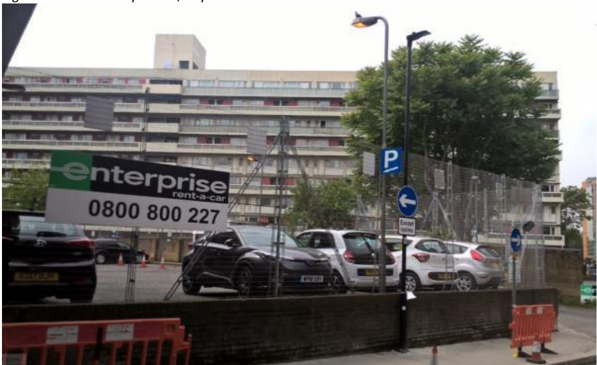
Figure 11 - Rear of Canterbury House as viewed from Upper Marsh
