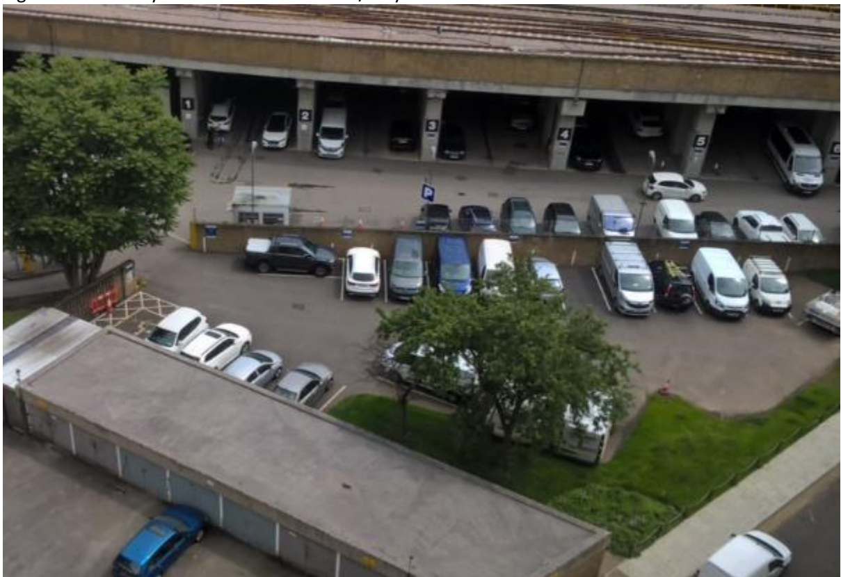
Figure 13 - Railway Viaduct at rear of Canterbury House
