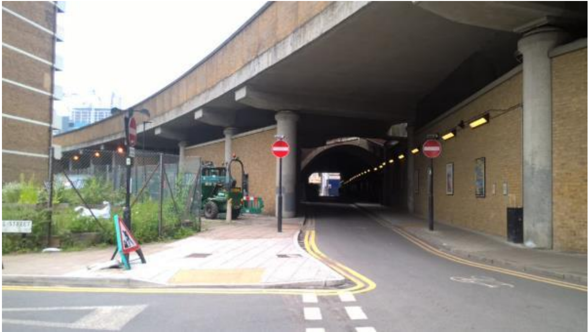
Figure 12 - Railway viaduct at Carlisle Lane / Royal Street intersection.
