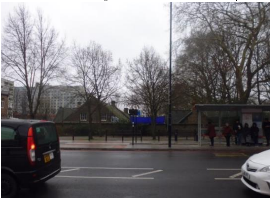
Figure 7 – former Christchurch School as viewed from the western side of Lambeth Palace Road
