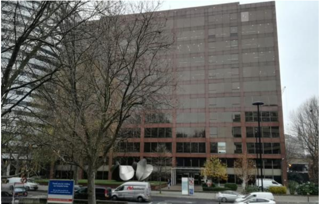
Figure 8 – Beckett House, Lambeth Palace Road
