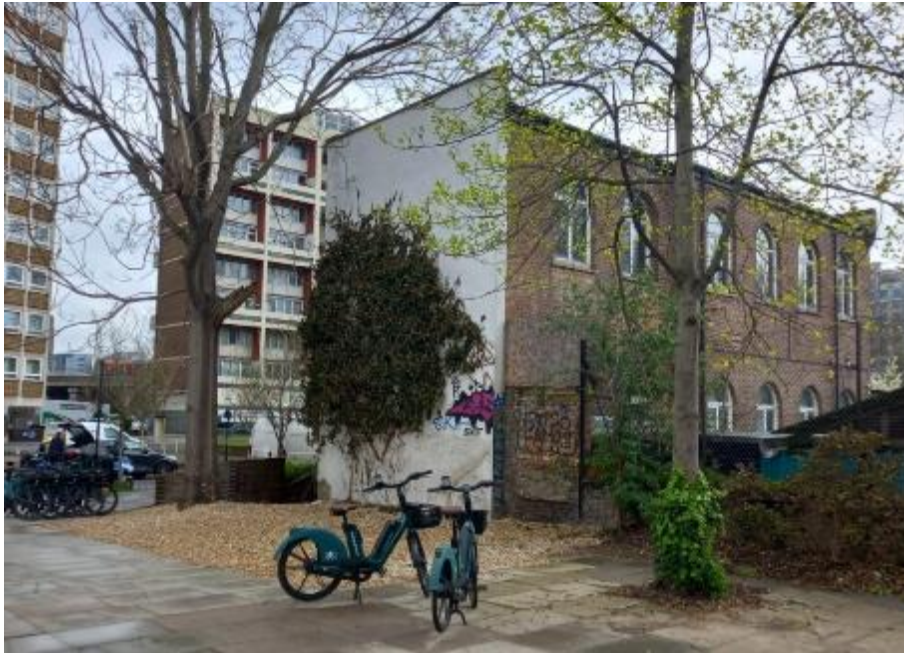
Figure 4 – No. 10 Royal Street’s flank to Lambeth Palace Road
