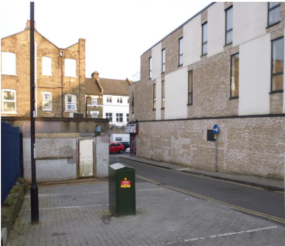
Figure 7 - Waylett Place looking towards Norwood Road
