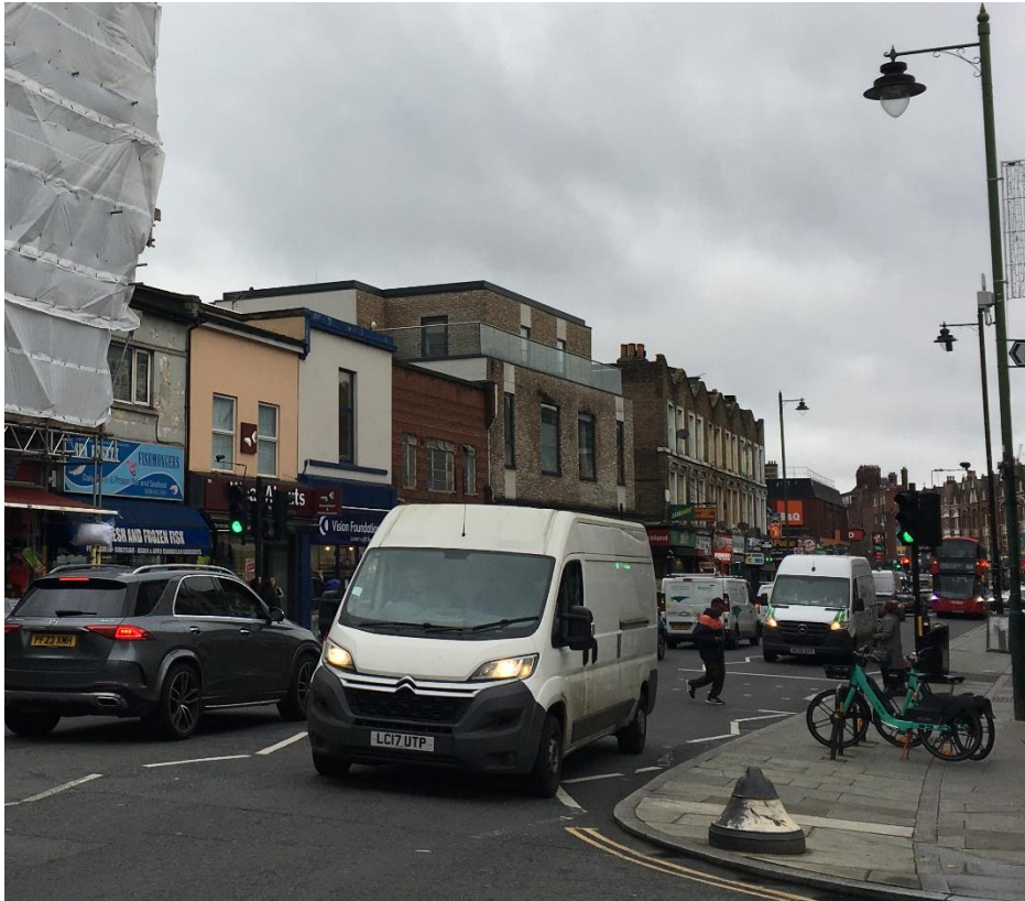
Figure 6 - The architectural quality of buildings on the site is generally low to average.
