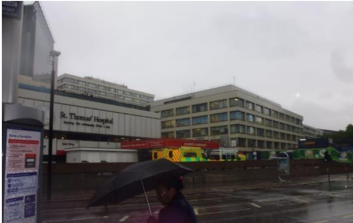
Figure 4 - A&E building and Lambeth Wing as viewed from Lambeth Palace Road. The viewer is within the Lambeth Palace Conservation Area.
