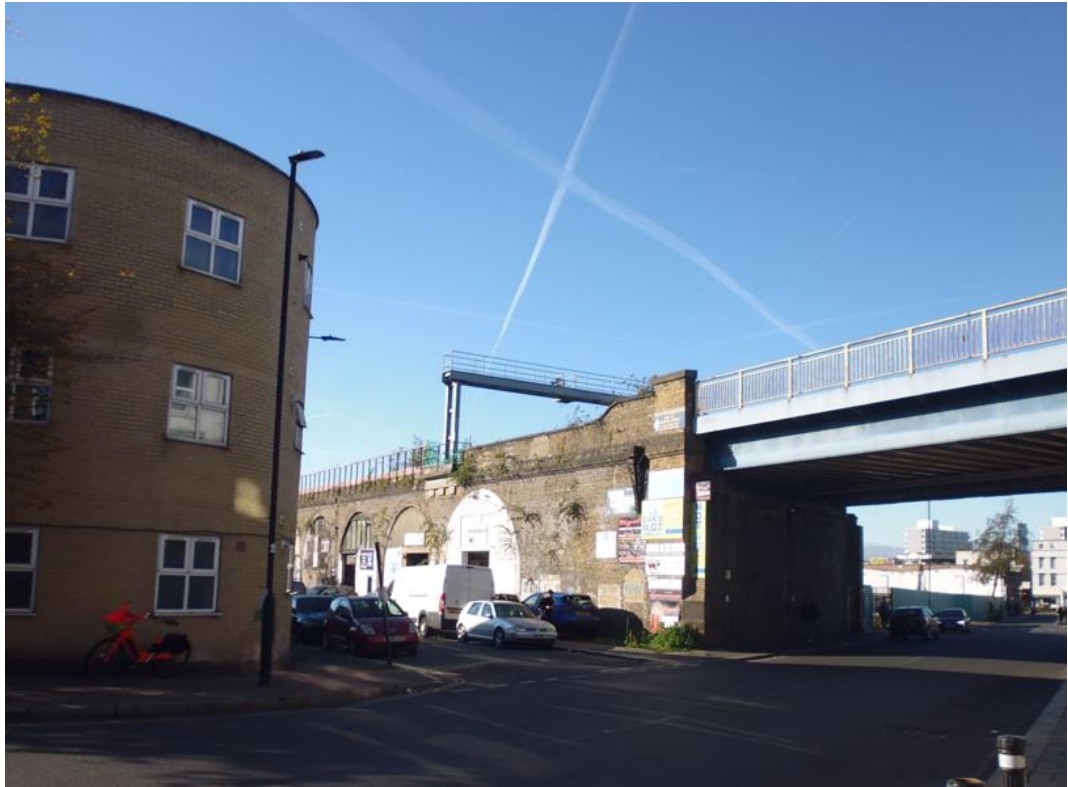
Figure 6- Corner of Hardess Street from Herne Hill Road.
