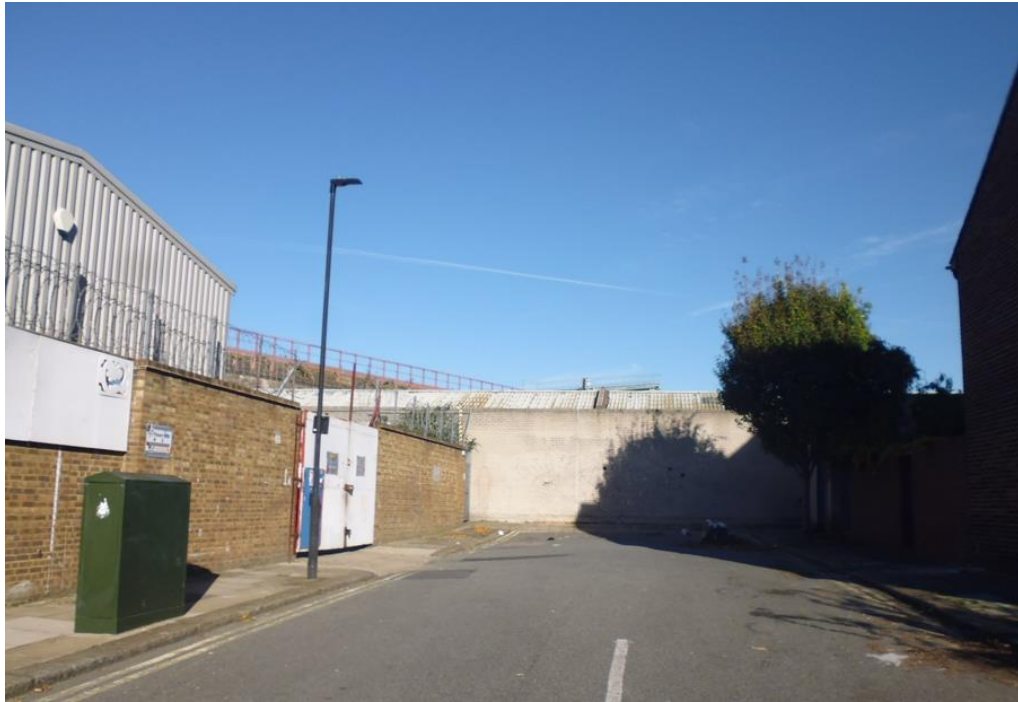
Figure 4- Wellfit Street dead end
