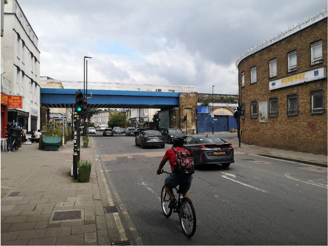
Figure 4 - View north along Coldharbour Lane with the site on the right.
