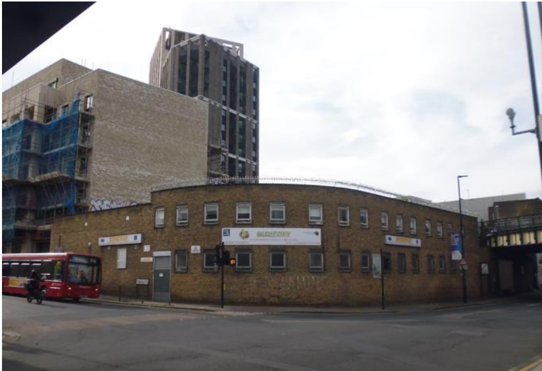
Figure 2 - The Sureway Church premises on the site.
