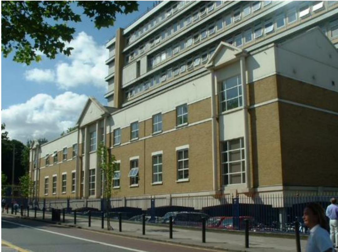
Figure 4 – The architectural quality across the campus lacks coherence
