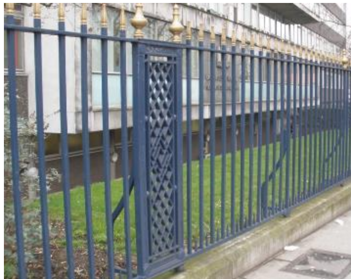
Figure 9 - The railings gates and piers to Denmark Hill (local list) are retained.
