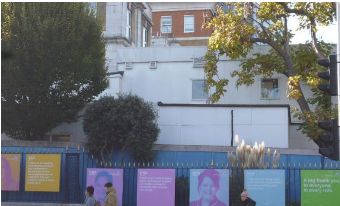
Figure 5 – Prefabricated buildings occupy prominent location on the Denmark Hill frontage
