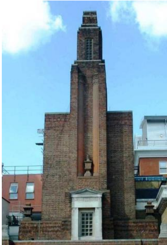
Figure 10 - The frontage block of the Guthrie Wing (local list) is retained.
